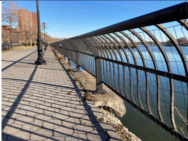
Photo 3: Typical Railing near 105th th Street looking north. Concrete is deteriorating under the rails. Balusters in background are not attached to anything as the concrete is missing
