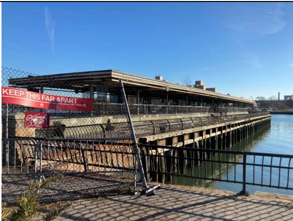
Photo 4: Pier at 107 th Street: See "C" on Keymap Potentially at major destination, it has deteriorated and been deemed unsafe and closed.
