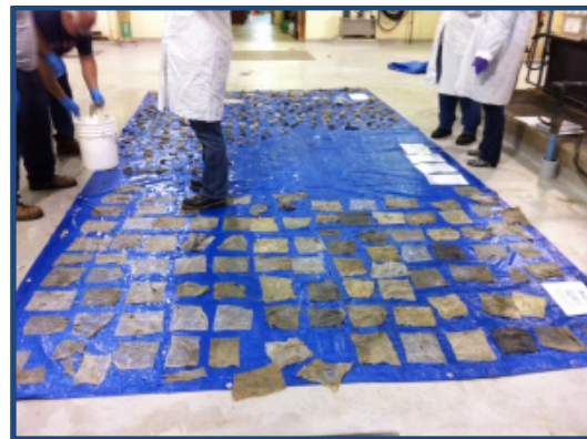
Materials removed during two hours of flow into the pump station, sorted to separate baby wipes (foreground) from other materials (background). Pre-campaign
