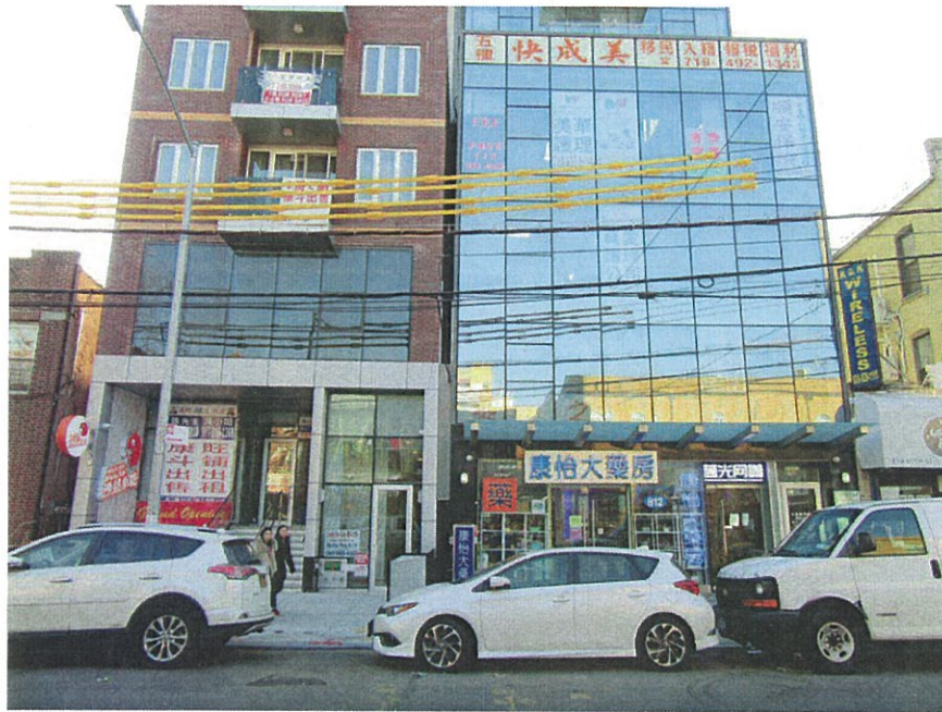
4. View of the Project Area facing southwest from 60th Street.
