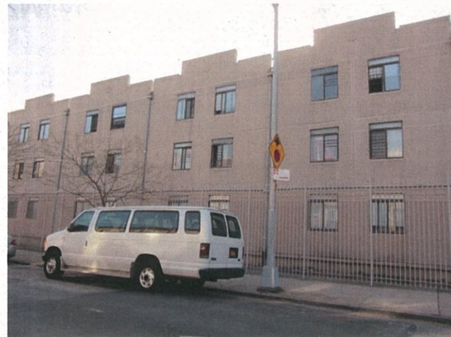
View of shelter from Hinsdale Street
