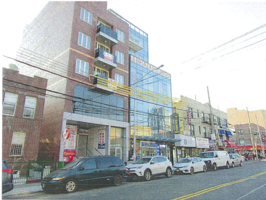
3. View of the Project Area facing west from 60th Street.
