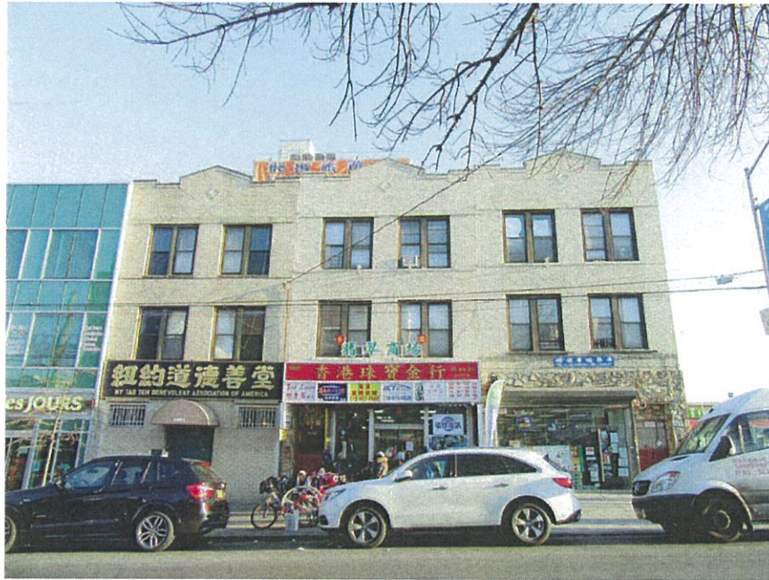
10. View of the Project Area facing southeast from 8th Avenue.
