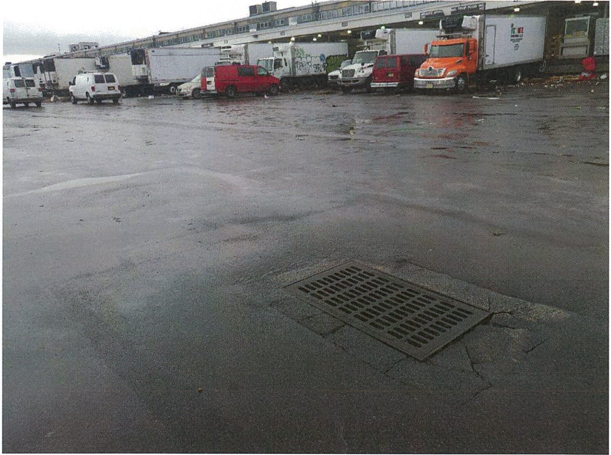
Catch Basin at Row B, cracking and depression
