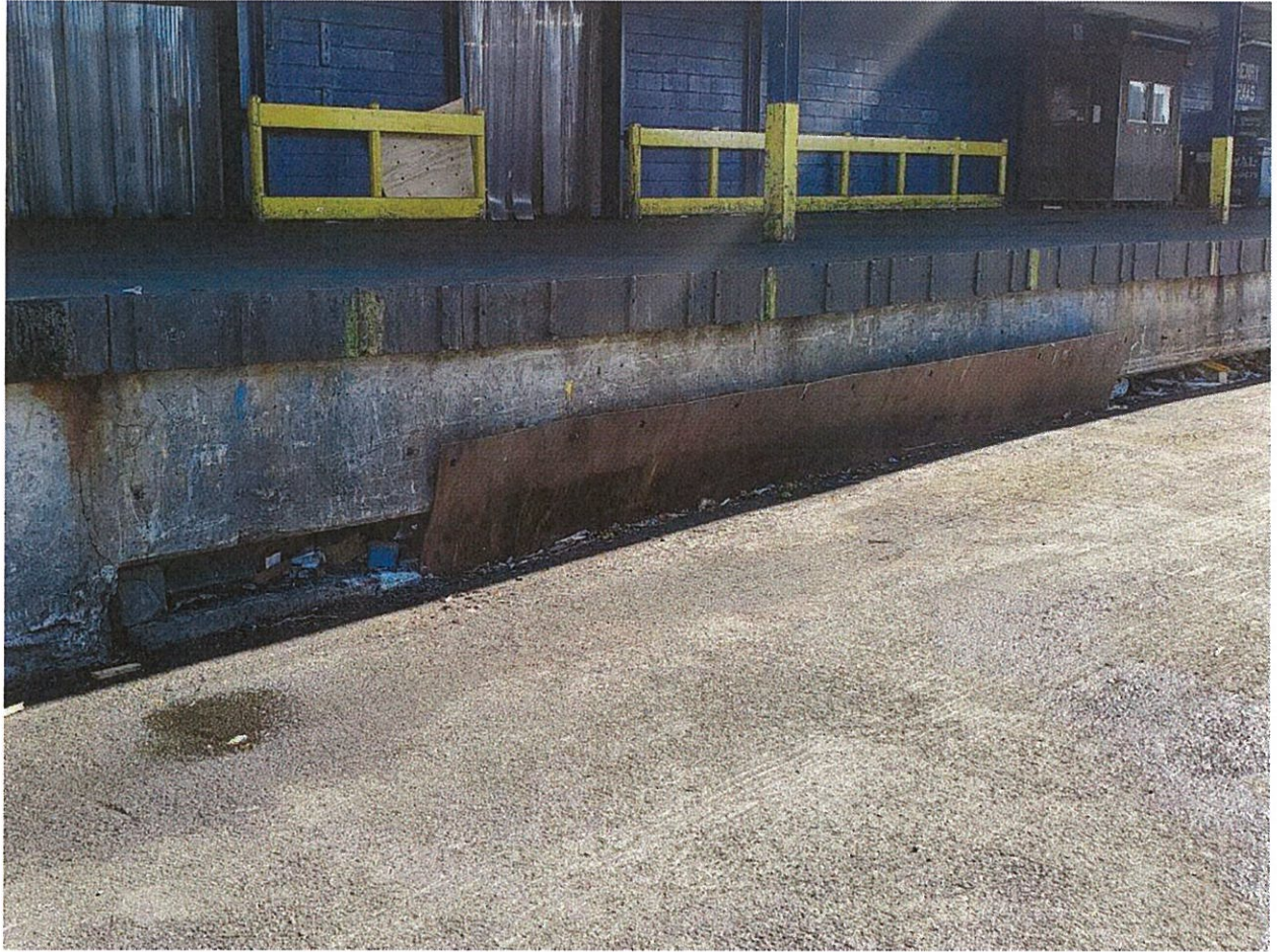
Dock Voids – temp steel plate to avoid further damage
