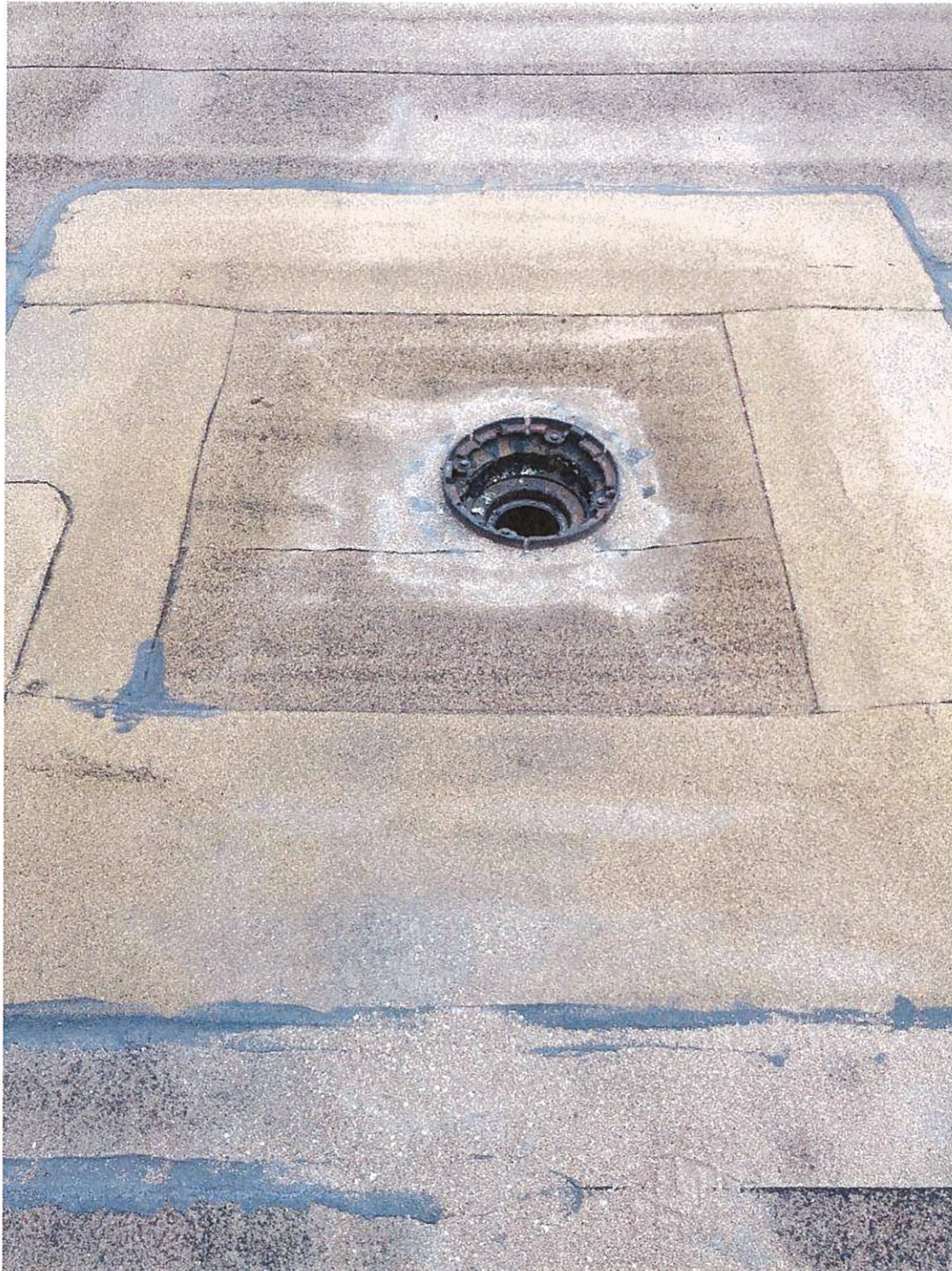
25 year old roof in need of repairs, storm caps missing, detrimental to our Food Safety Plan
