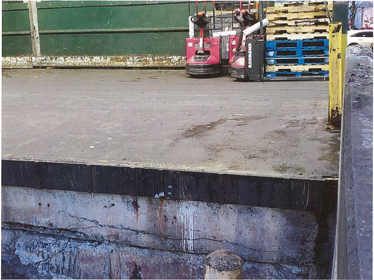
Cracking and deteriorating voids in dock
