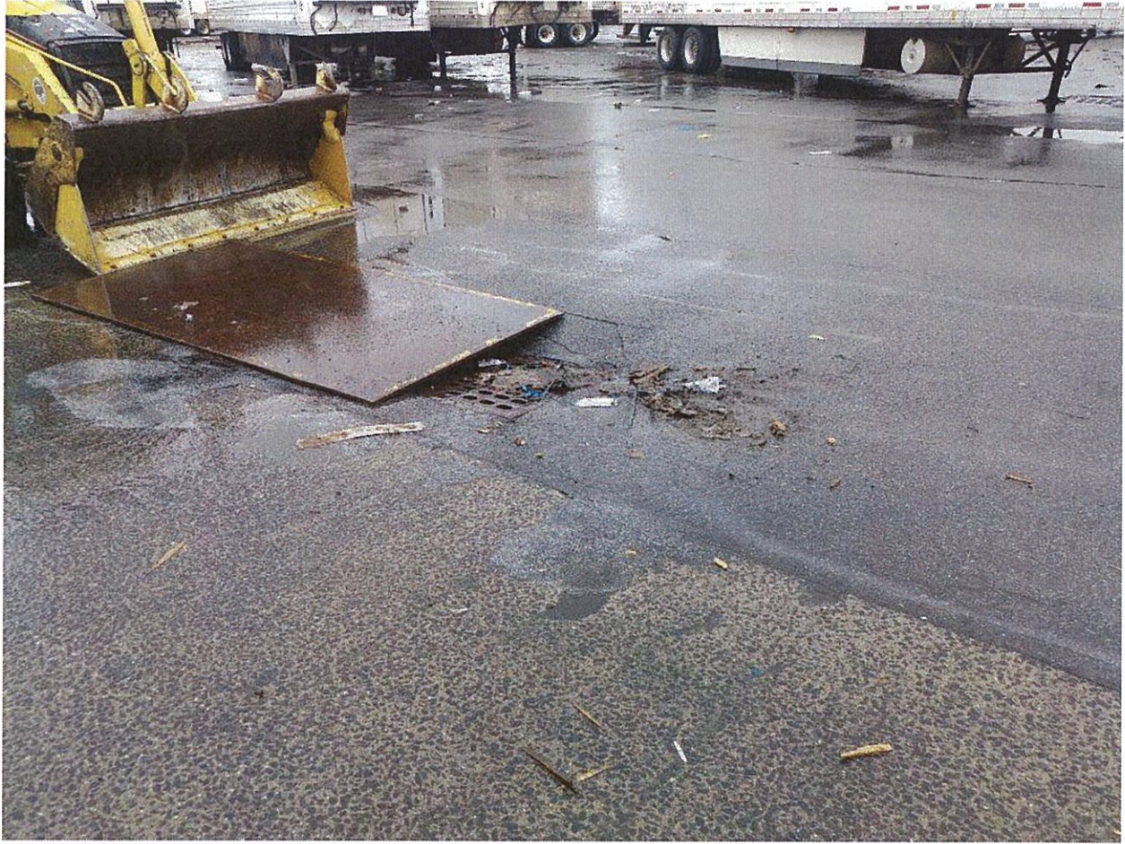
Dock plate used to avoid depression in street from collapsing roadway at drain point
