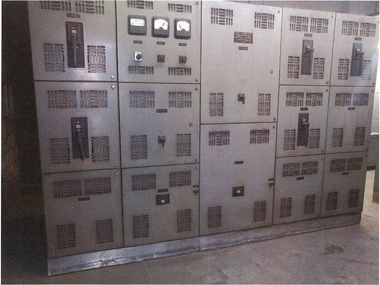
Aging out Market Equipment for Electrical Vaults
