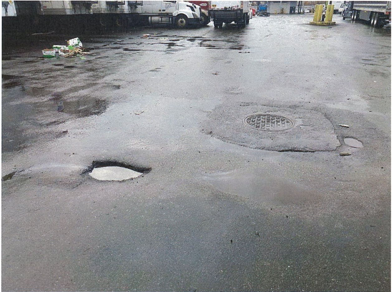
Pot holes Row B, cracking and failing of sewer cement
