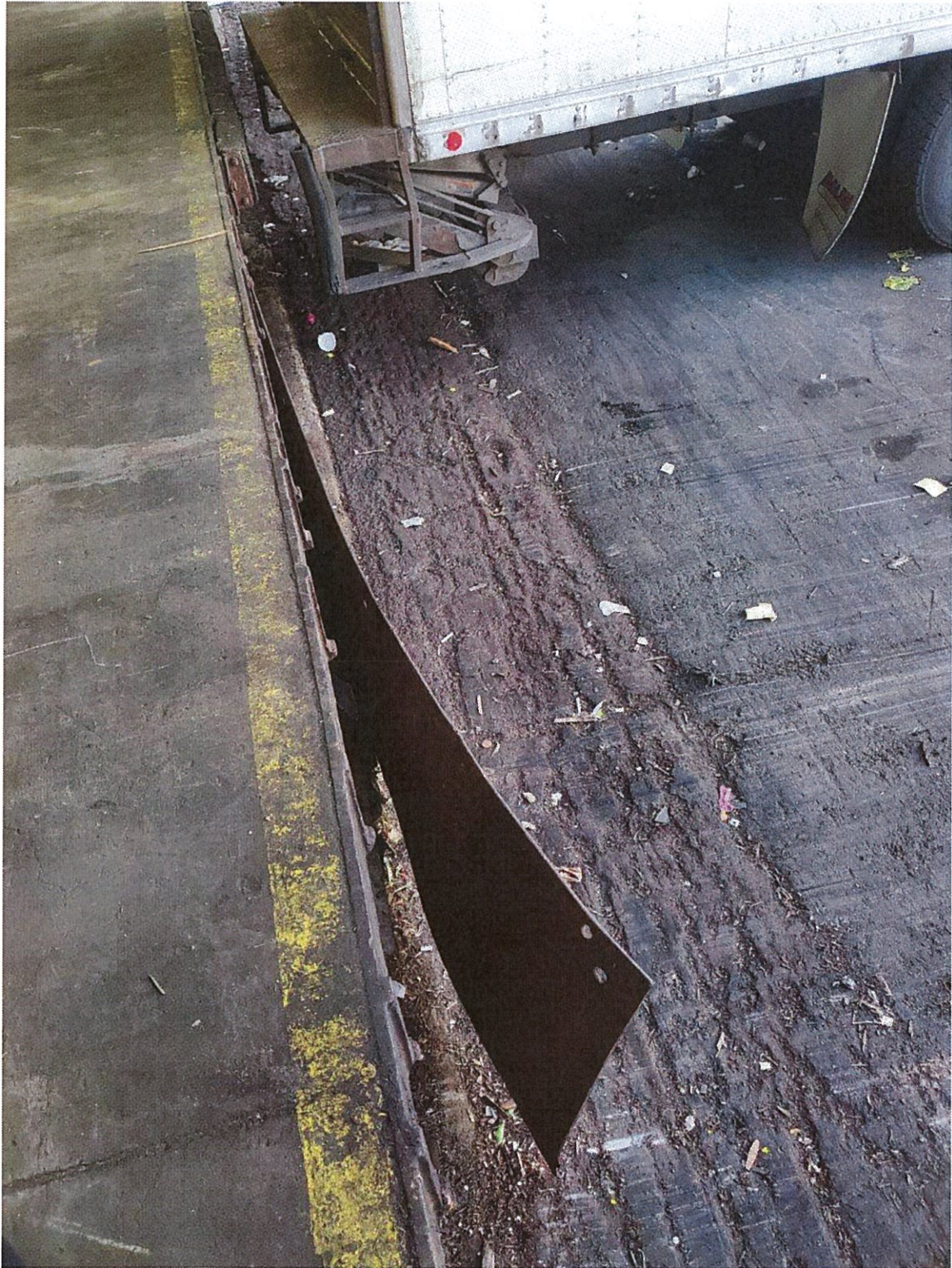
Temporary steel plates - dock side
