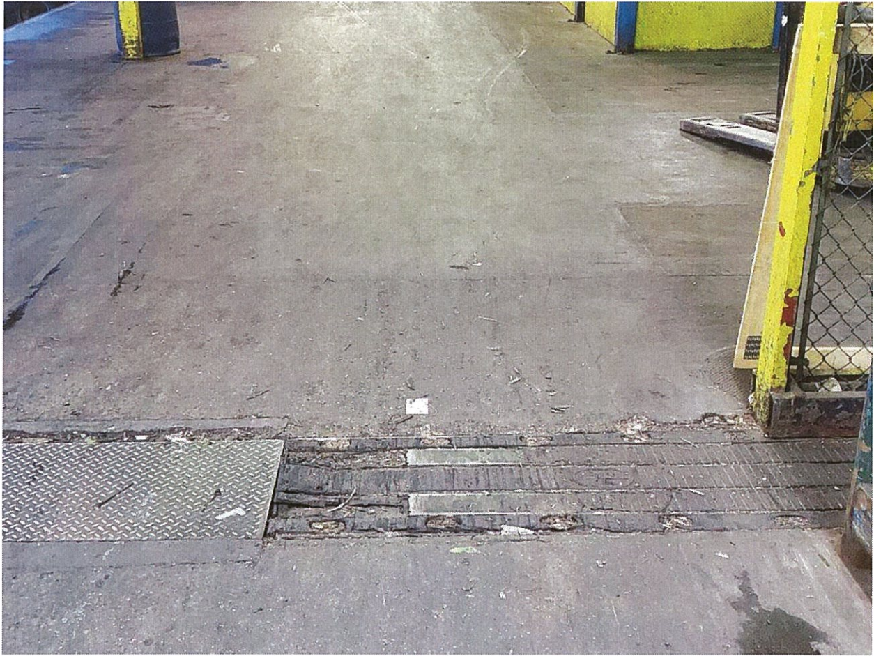
Expansion Joint Row B (various locations)
