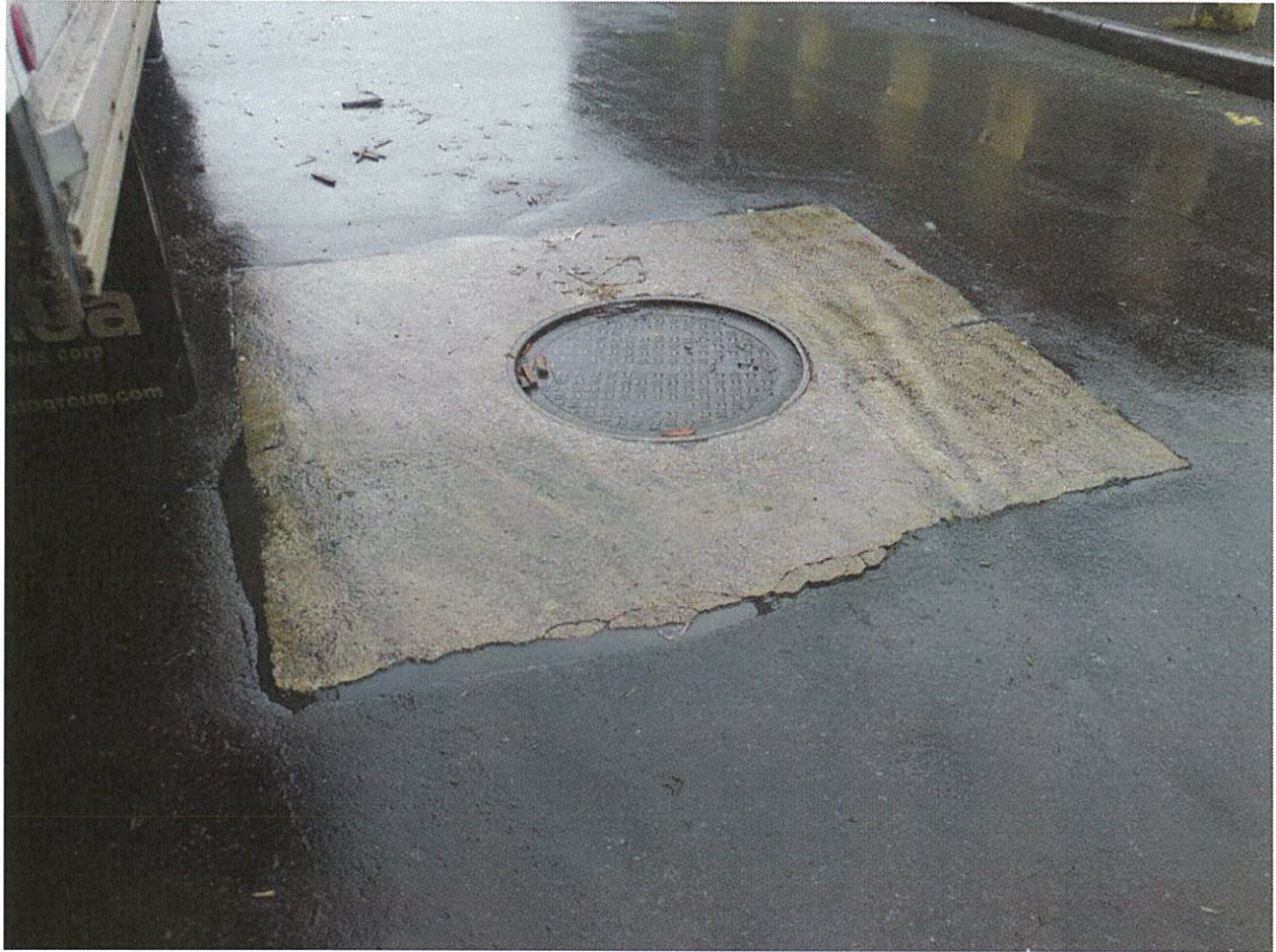
Cement around the sewer is cracking and failing
