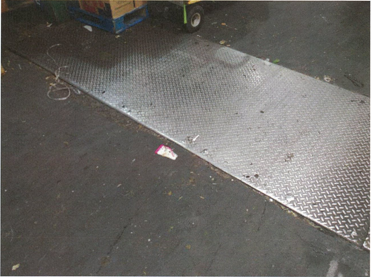
Repaired Expansion joint Row B
