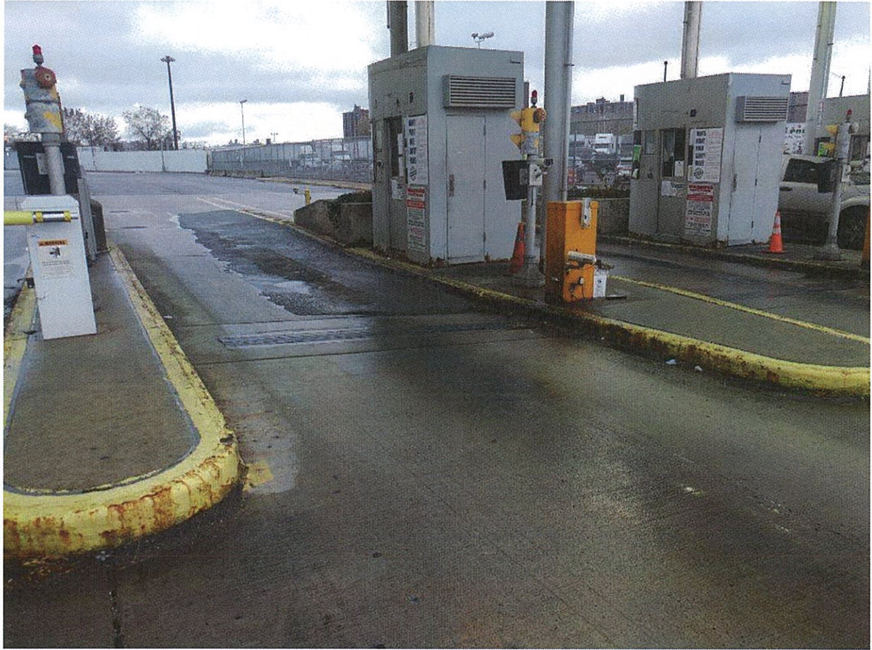
Lane 2 depression and incline causing vehicles to come into contact with booth
