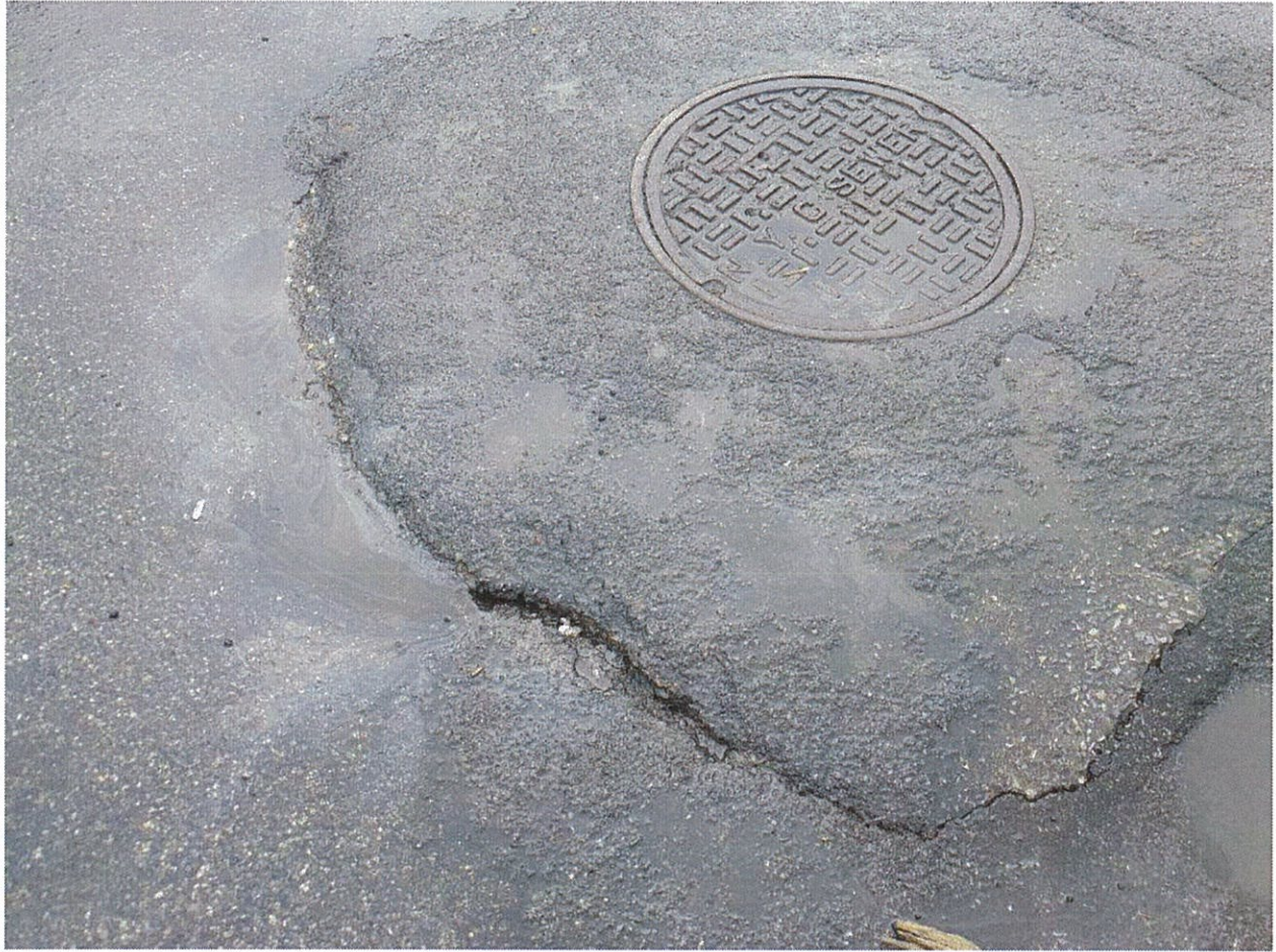
Pot hole at Row B, cement failing around sewer
