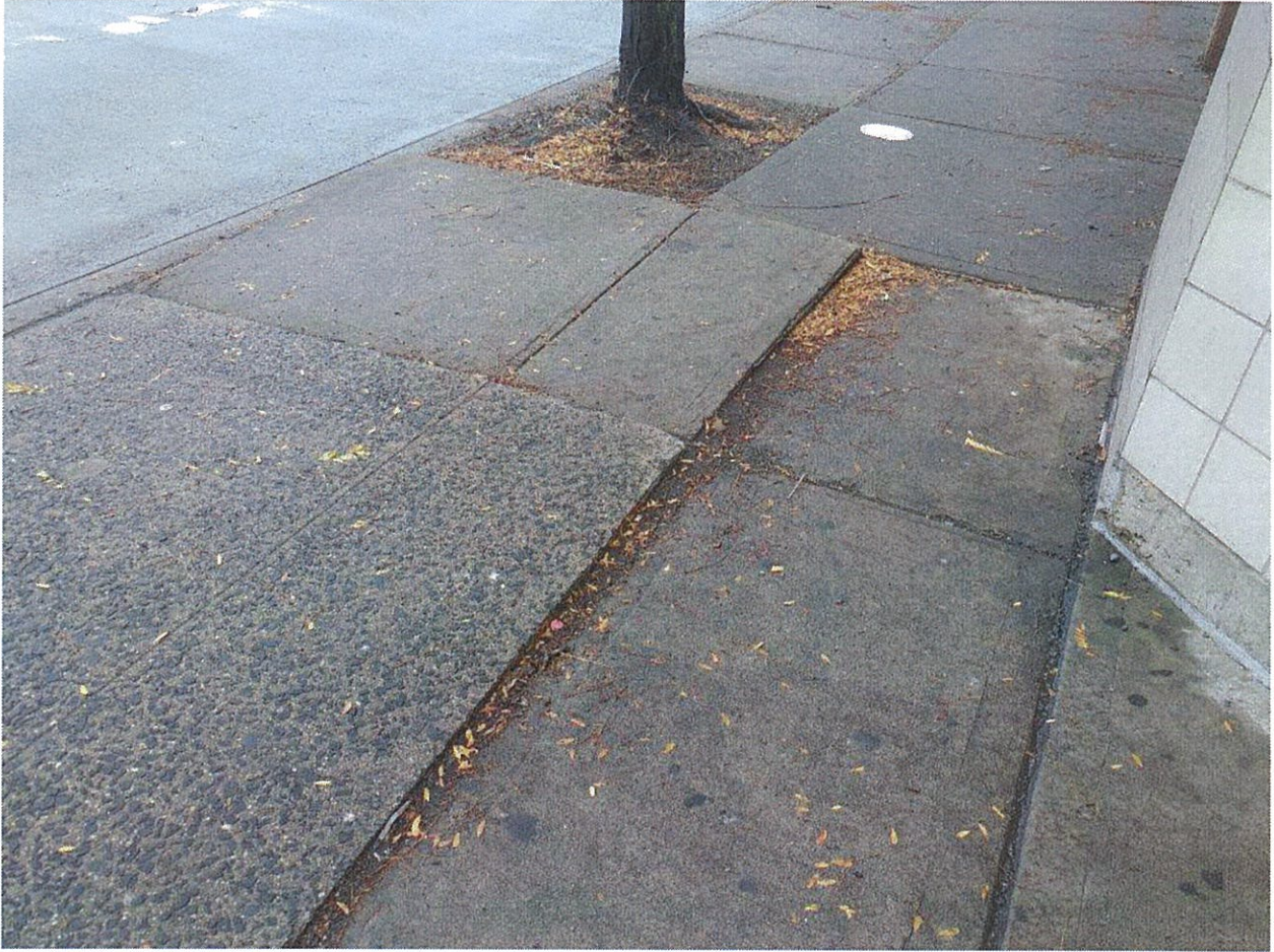
Sidewalk at Bust stop on Halleck Street, tree roots pushing up sidewalk
