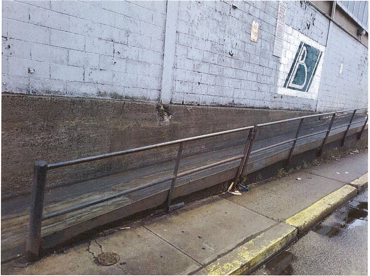
Row B street ramp in need of replacement, rails failing, paint chipping
