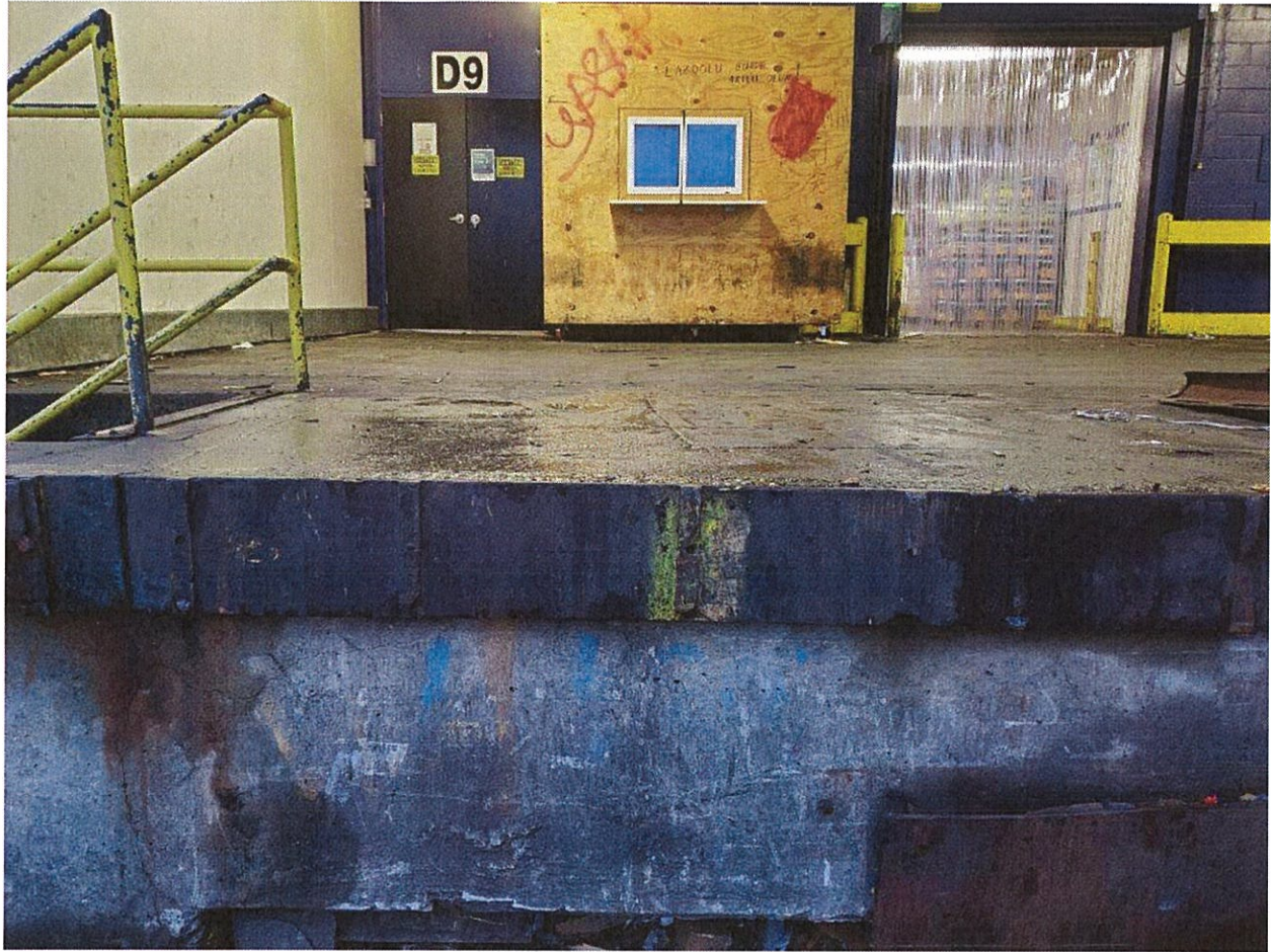
Deterioration of Platforms – major Voids
