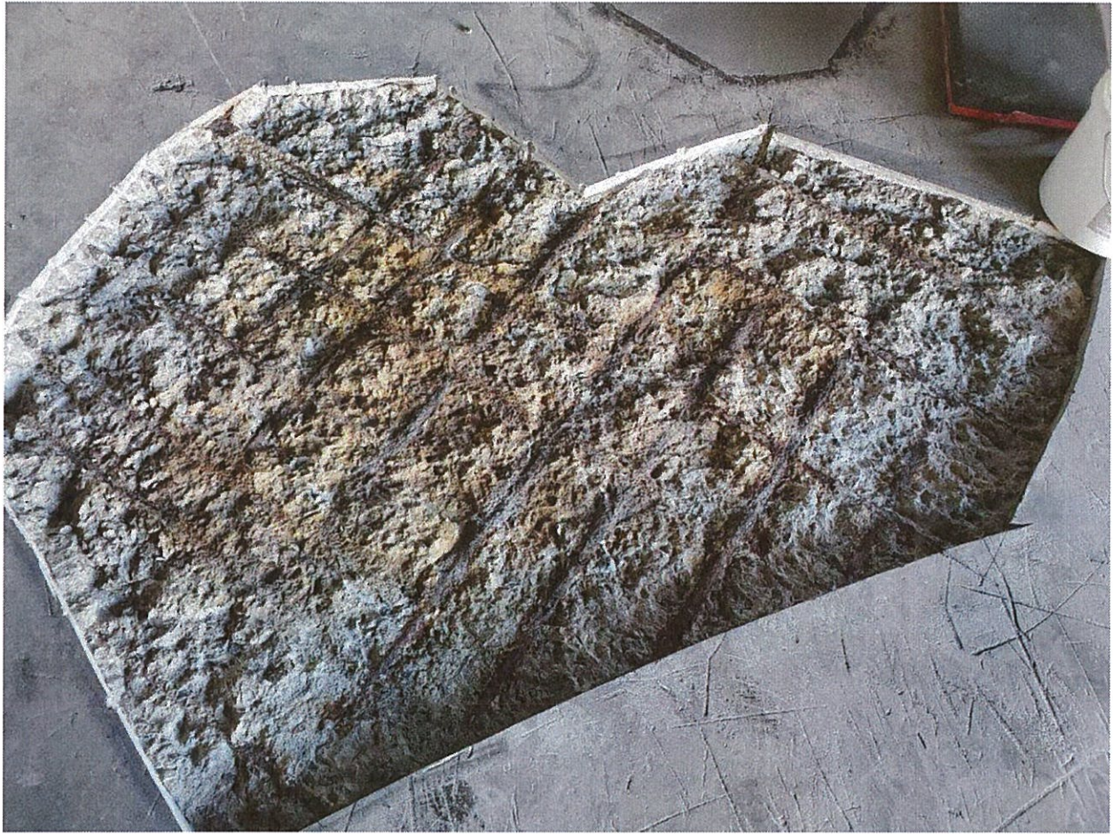
Docks deteriorating - prepping for epoxy filling
