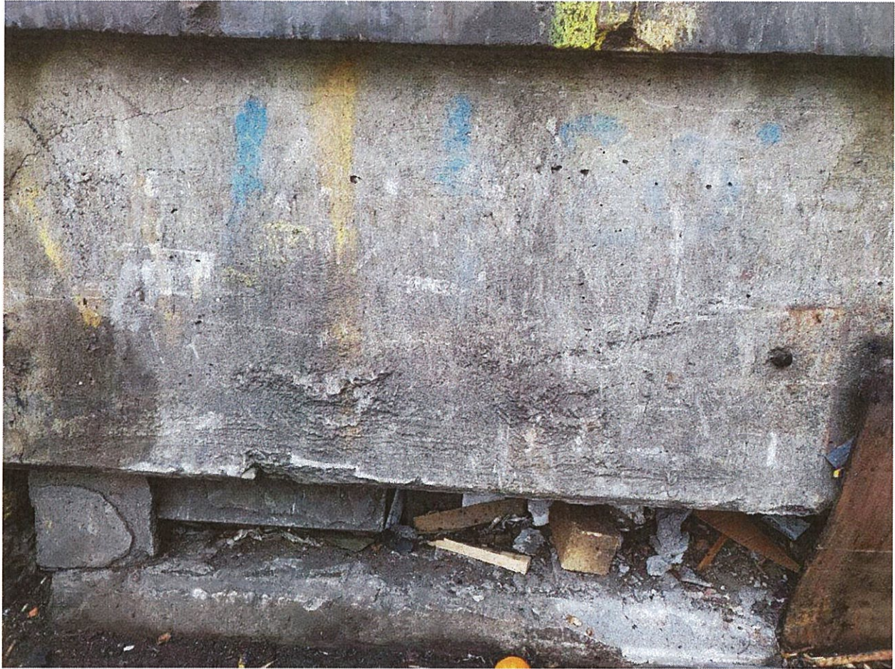
Voids underneath the platform (various locations)
