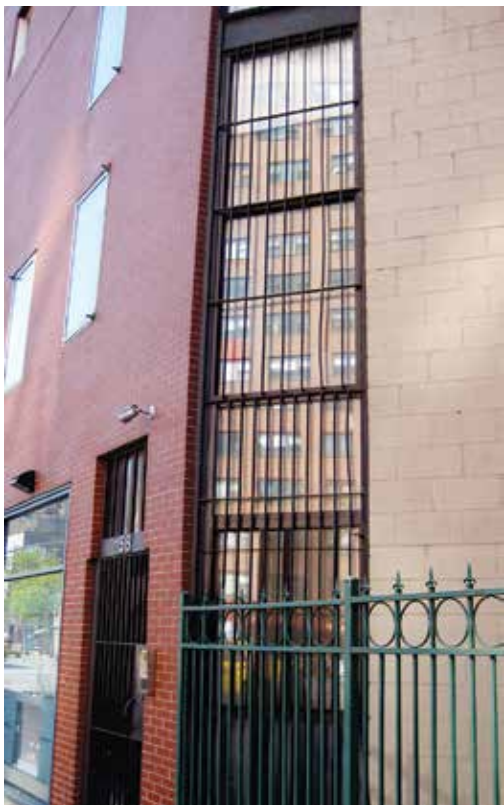
This security grille creates a pattern that will deter birds from flying to reflections. Photo by Christine Sheppard, ABC
