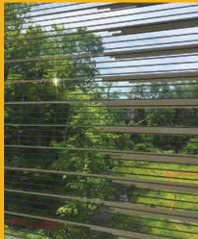
Glass detail, showing frit pattern
