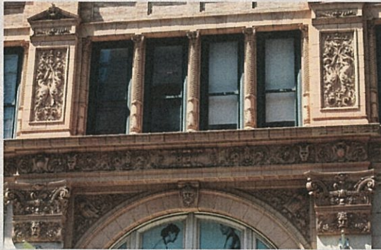
Terra-cotta detail, LPC 2018
