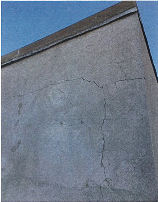
Cracking facade at Central Library, Brooklyn
