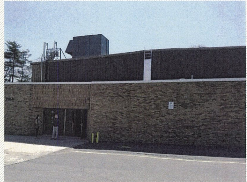
Main Entrance to Gymnasium
