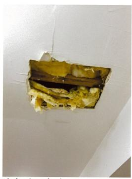
Moldy insulation & rotting beam August 5, 2018 at 10:27:46 AM
