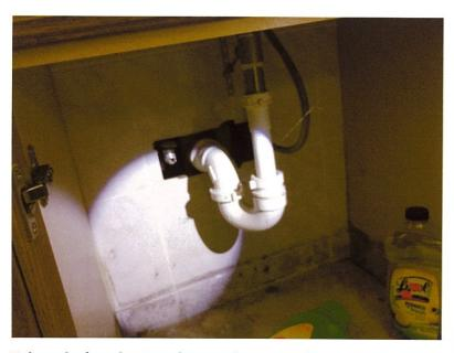
Taken during the HPD inspection.. No violation? Missing pipe, mold, open unsealed around pipes, rat enterance, rotting
