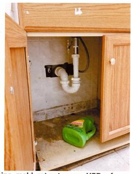
Missing pipe, mold, rat enterance HPD refuses to write a violation.
