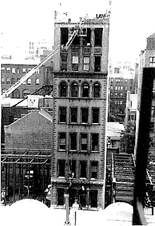
30 Great Jones Street during demolition
