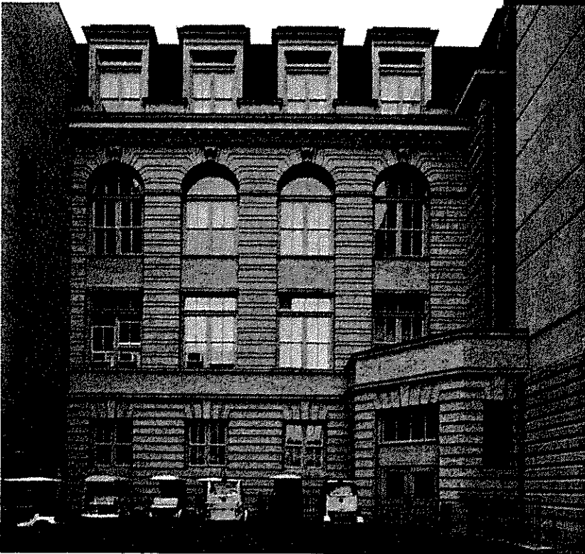
Museum (now Library) Building, New York Botanical Garden, rear (east) facade
