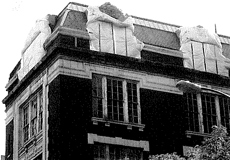
After: Removal of Architectural Features
