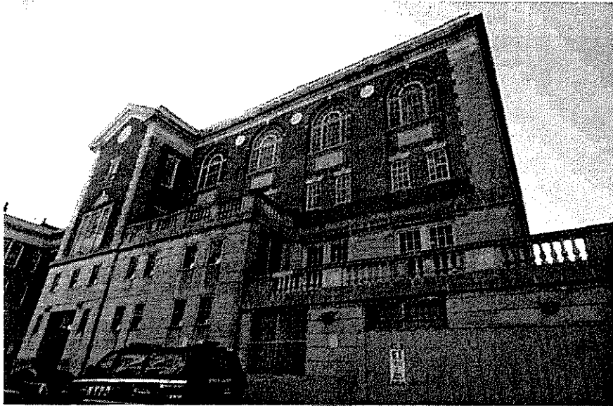
Jamaica High School Central rear wing, east façade Photos: Christopher Brazee, 2008
