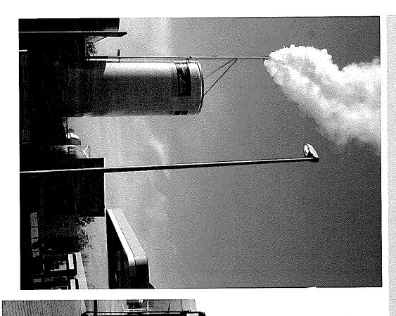
35 and 70MPa, LH2 dispensing 900 bar Pipeline (1.5 km) & local LH2 Storage
