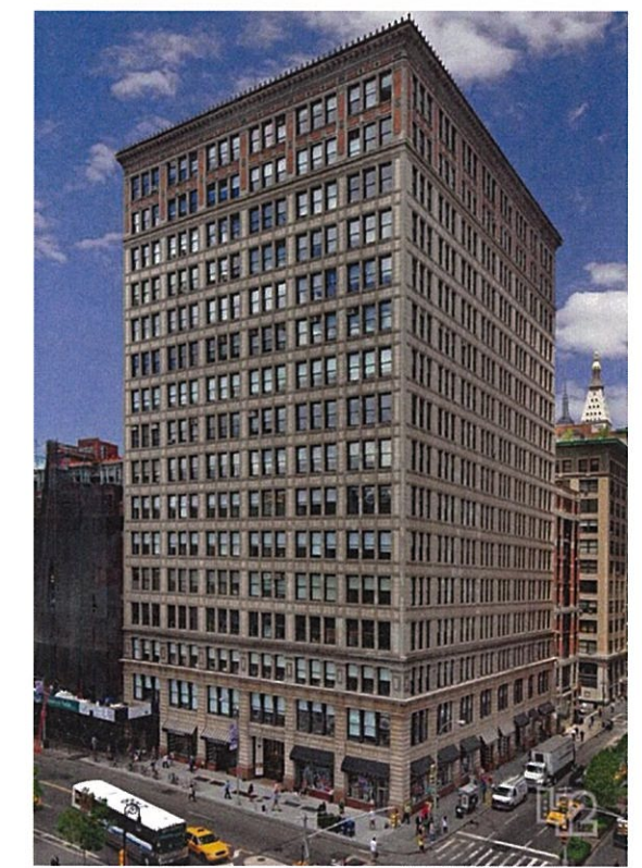
(E) EVERETT BUILDING
