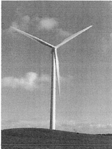
Example of a Horizontal-Axis Wind Turbine
