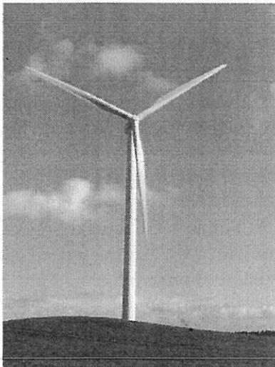
Example of a Horizontal-Axis Wind Turbine
