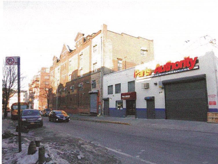
15. View of the east side of Franklin Avenue facing northeast.
