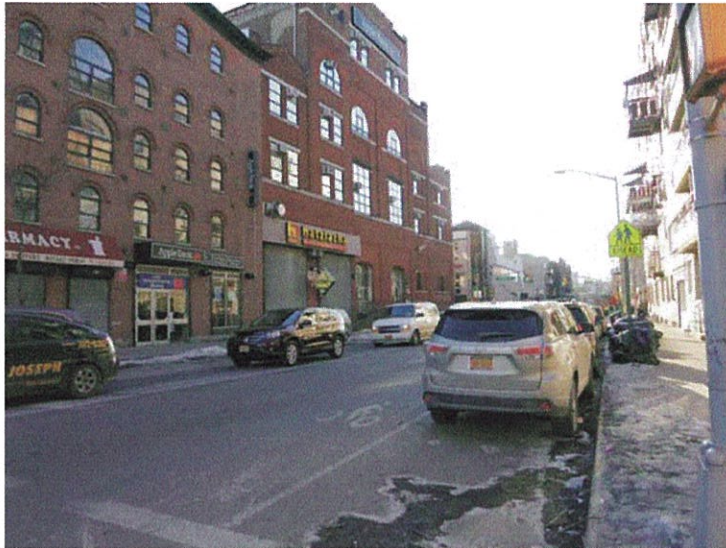
10. View of the south side of Flushing Avenue facing southwest.
