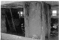
Condition of the steel H-piles with severe corrosion and knife-edged flanges
