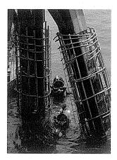
The repair methodology consists of applying an outer concrete jacket over a deteriorated steel pile and reinforcing most piles with rebar to restore the piles structural capacity. It will take approximately four to 5 years to complete pile restoration, since most work is done by divers in the water. Courtyard fields are not expected to be impacted other than the need for access along the edges.
