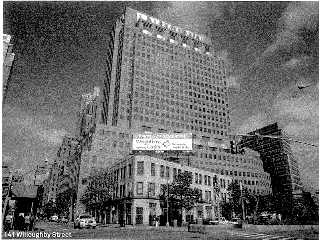
1 VIEW OF SITE, FACING NORTHWEST FROM FLATBUSH AV. EXT. AND WILLOUGHBY ST INTERSECTION.
