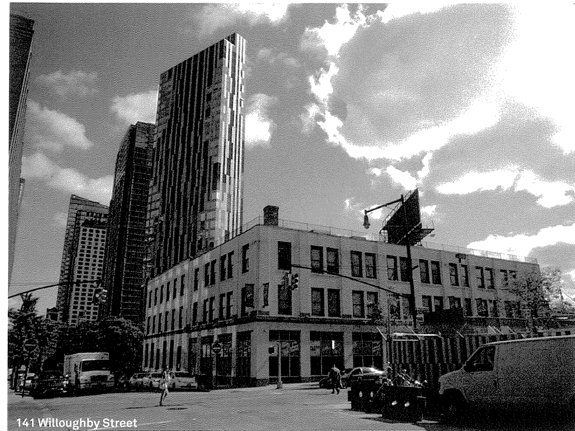
2 VIEW OF SITE, FACING NORTHEAST FROM GOLD ST AND WILLOUGHBY ST INTERSECTION.
