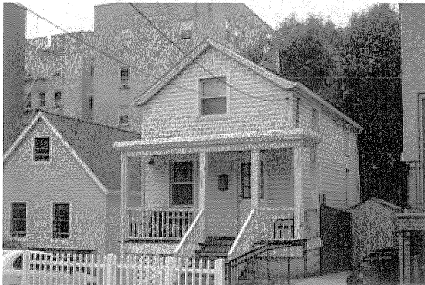
3. Looking south from E. 235th Street Photo taken: 6.19.15
