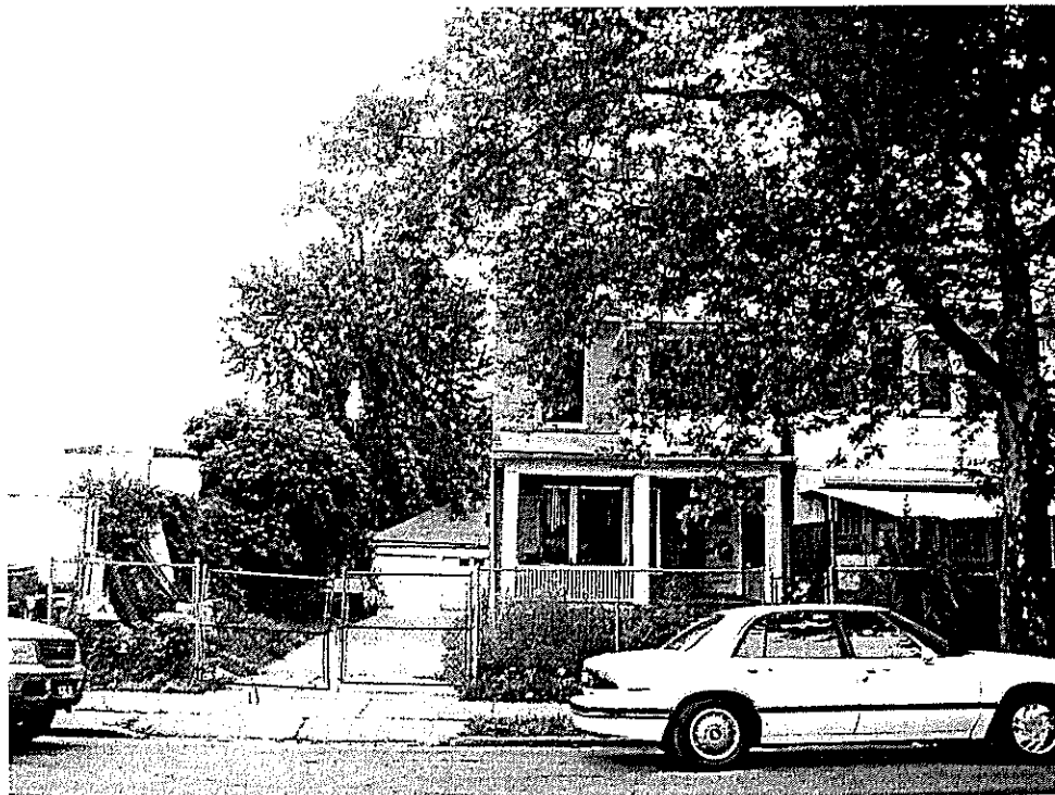
Photograph 2: View of Lot 8. Looking south from Turner Place.
