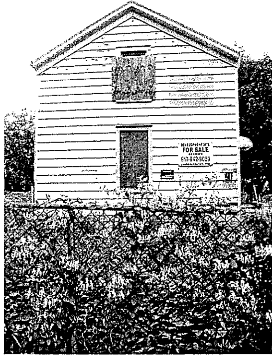
Photo 8-7: Vacant residence on southern side of project site, view facing north from Hinckley Place.
