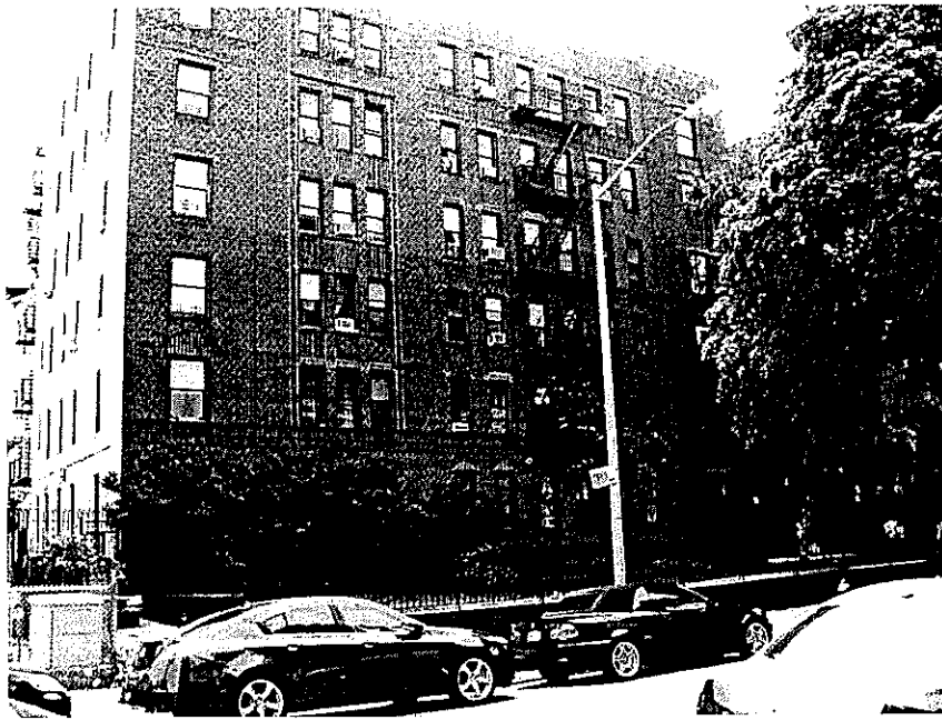
Photo 8-11: Six-story apartment building across Hinckley Place, facing south from the project site.
