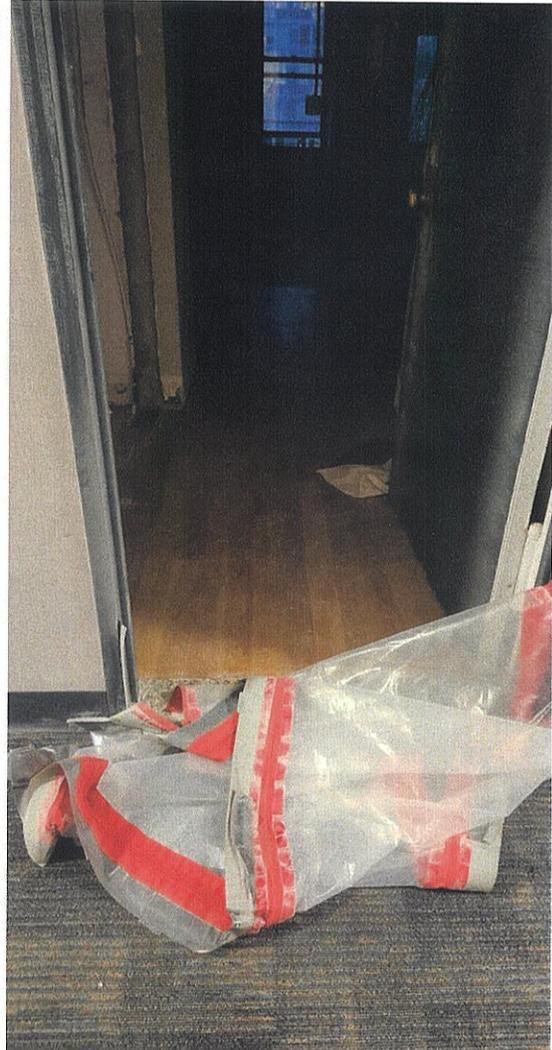
**788 Columbus Avenue Apt 5MN Being Frankensteined. 05152023. Apt Door left Wide Open in Violation of Construction Regulations. Protective Plastic Cover That Is Supposed to Cover The Entire Front Door On The Hallway Floor Permitting Dust With lead and Asbestos to Be Tracked and Filtered Throughout The Fifth Floor Hallway and Building.**
