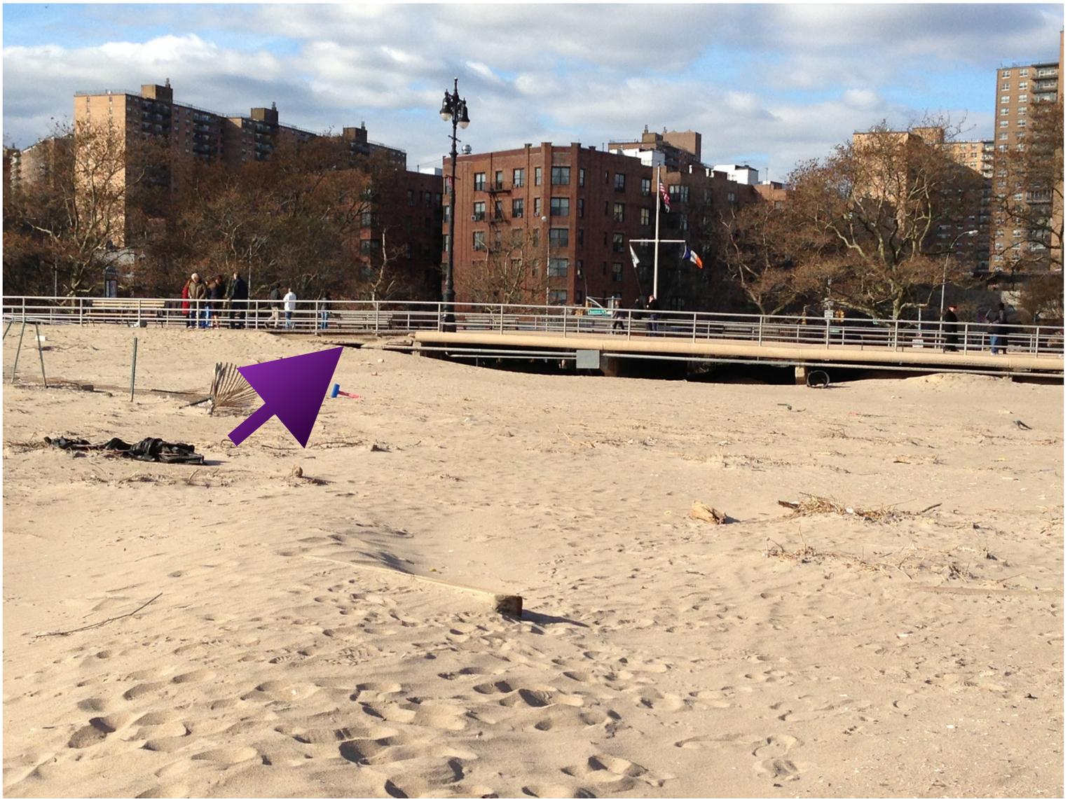
The line of demarcation is even more dramatic up close. The eroded area varied from 1-3 feet in height for the entire length of the concrete slab section, about three blocks.
