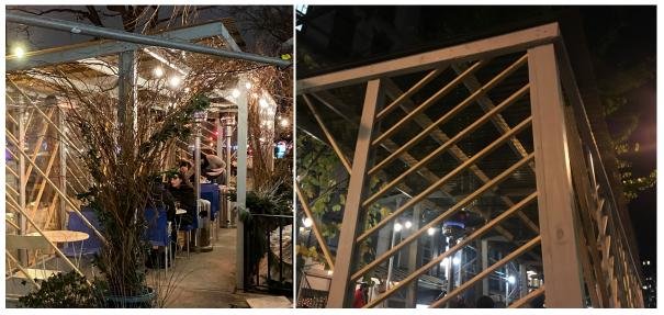
Propane heaters inside enclosure and placed within 12" of combustible materials (wood)
