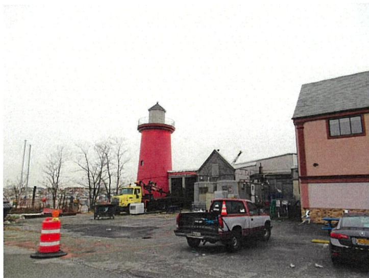
3. View of Development Site 1 facing northeast from Plumb 2nd Street.
