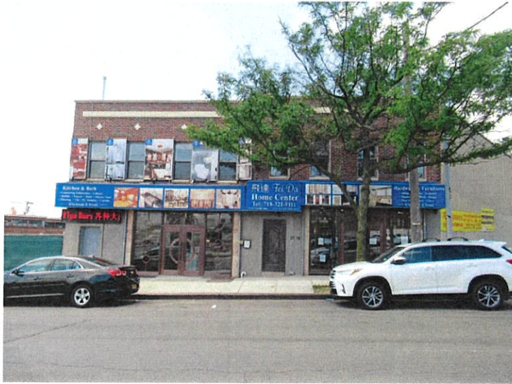
4. View of the Project Area facing west from College Point Boulevard.
