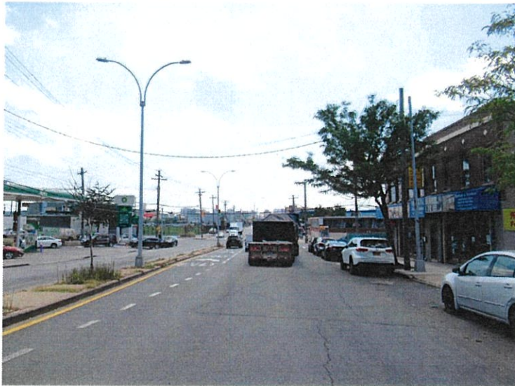
6. View of College Point Boulevard facing southeast (Project Area at right).
