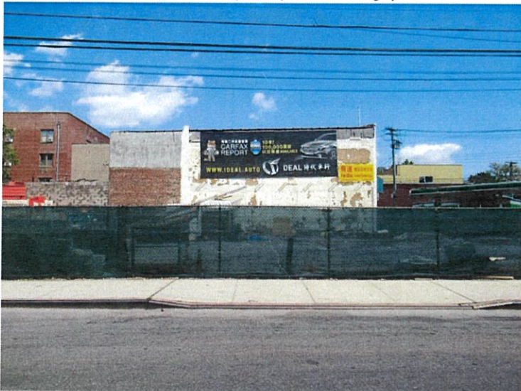
12. View of the Development Site facing north from 28th Avenue.
