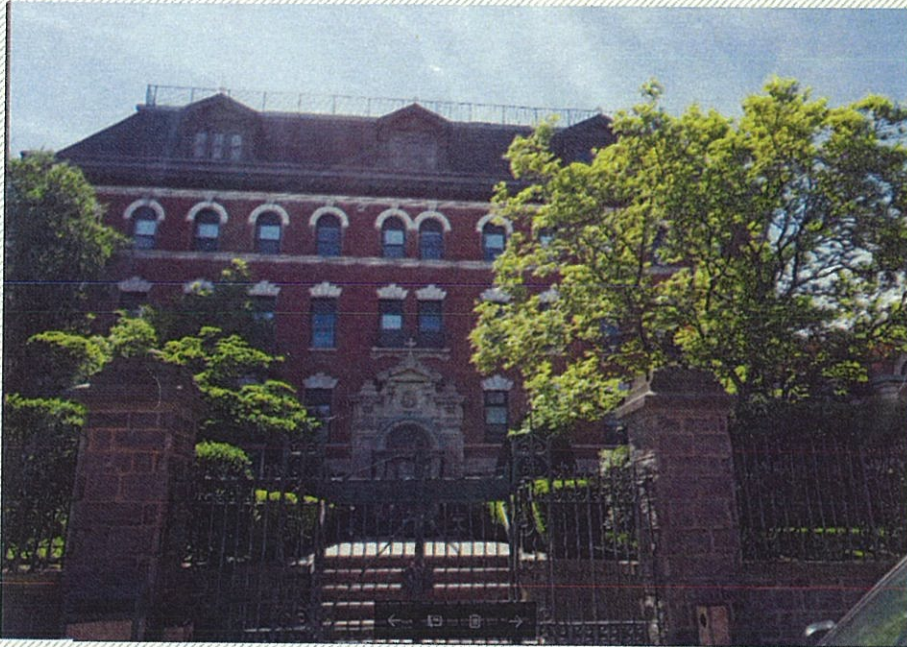
The former orphanage building viewed from 12 th Avenue (not included in Project Site, separate owner/developer)
