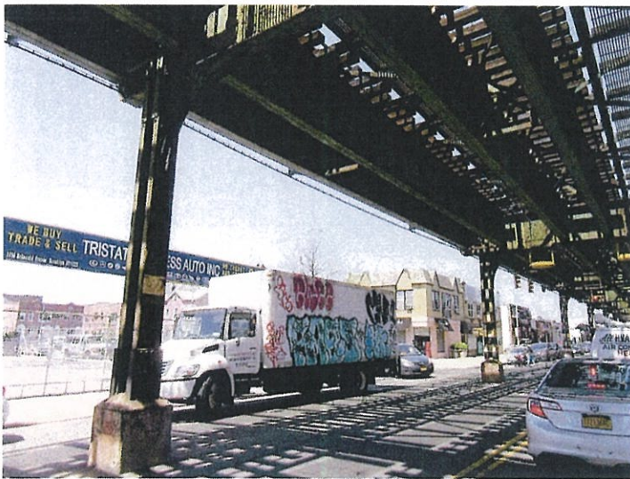
6. View of the west side of McDonald Avenue facing northwest from the Project Area.
