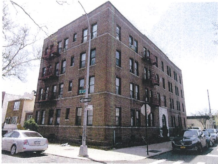
7. View of 14 Woodside Avenue facing southwest from the intersection of Woodside Avenue and East 2nd Street.
