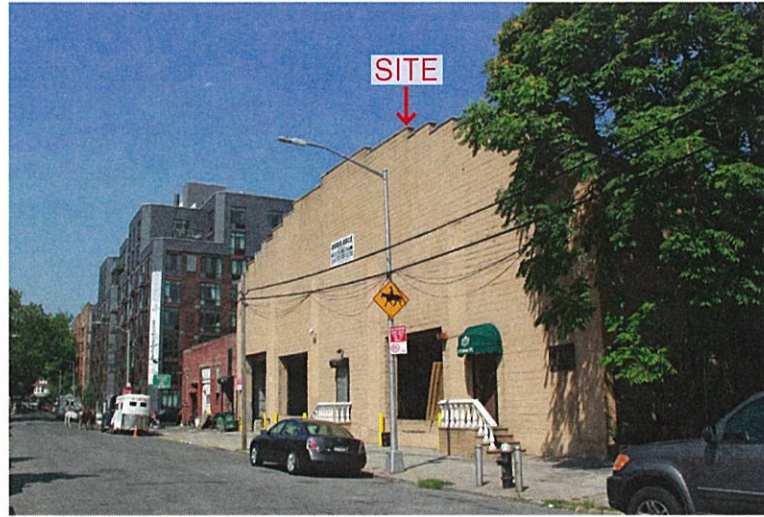
2 SW view on Caton Place
