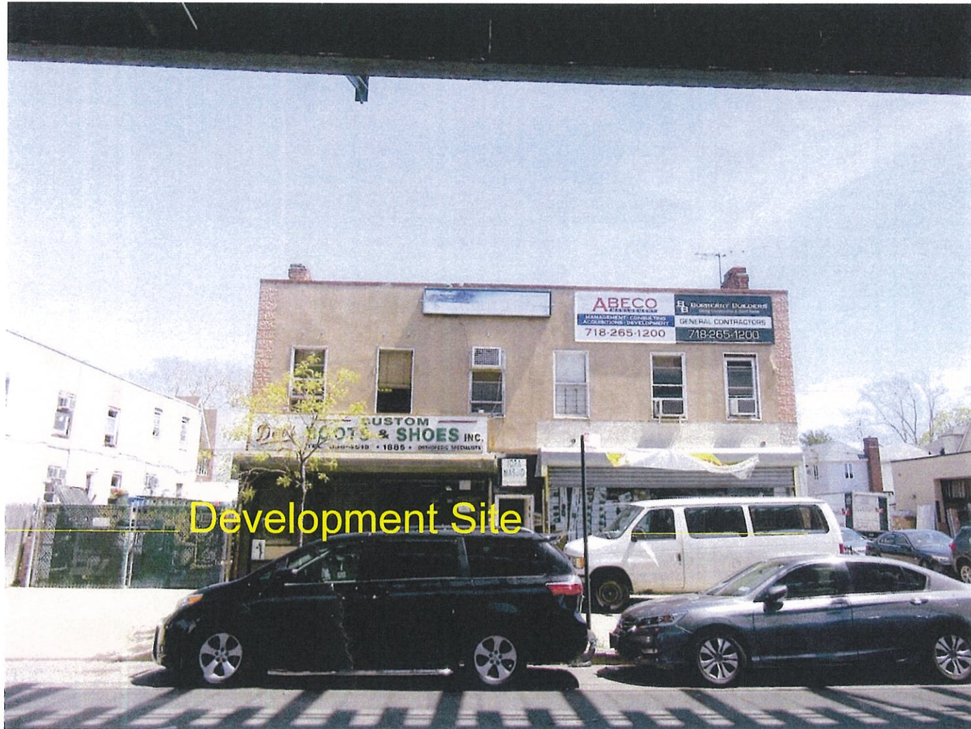
View of the Development Site facing east from McDonald Avenue.
