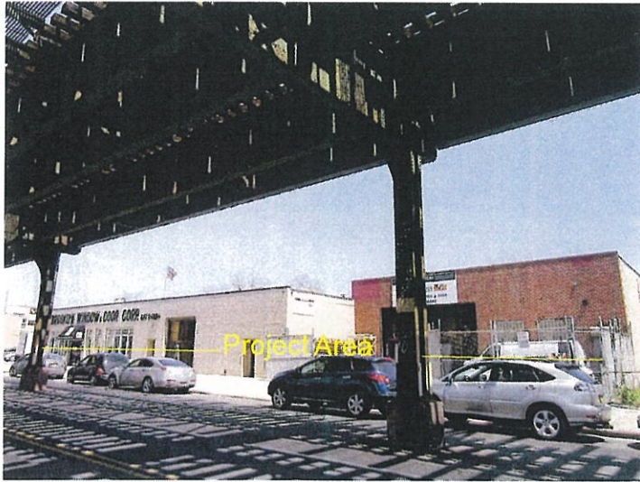
1. View of the Project Area facing northeast from McDonald Avenue.
