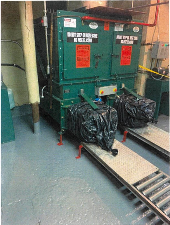
Newly renovated interior compactor room at Rutgers Houses
