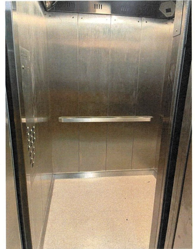
New elevators at Richmond Terrace
