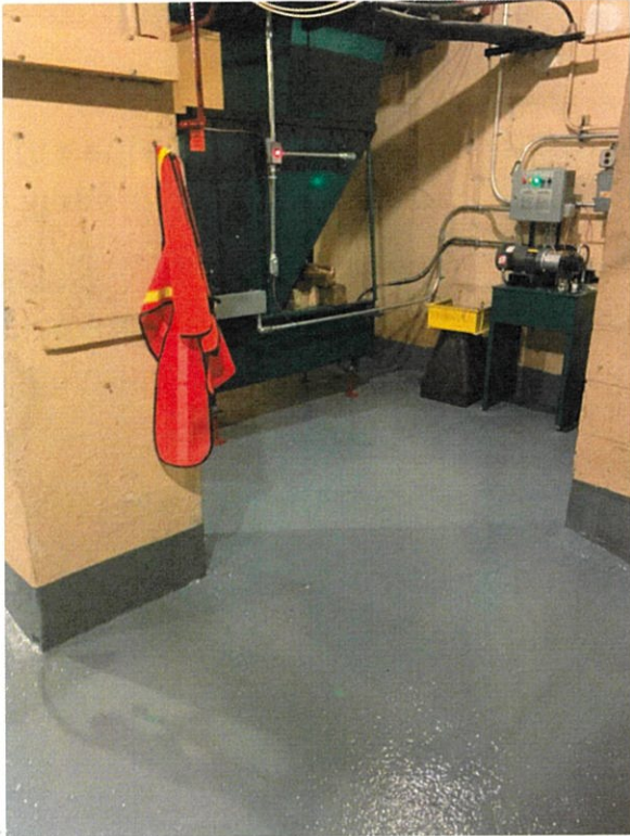
Newly renovated interior compactor room at Hernandez Houses
