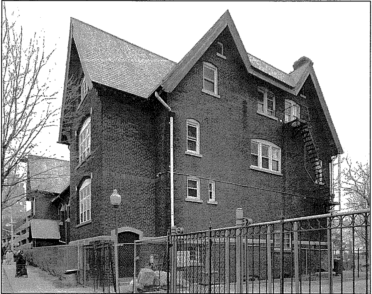
Grace Episcopal Church Memorial Hall West Facade Photo: Christopher D. Brazee, 2010
