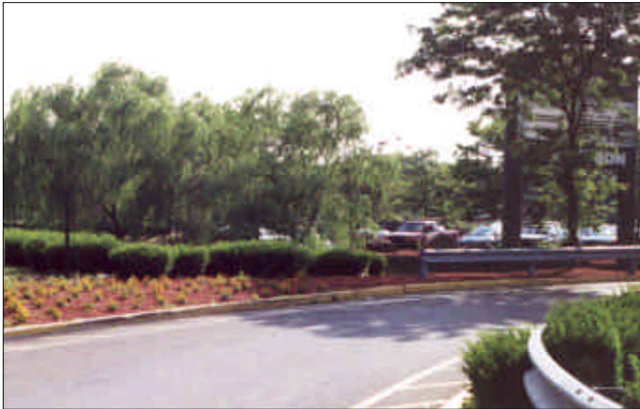
Entrance with landscaped detention basin and annuals in planting beds.
