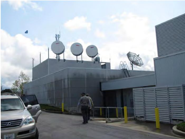
*Microwave dishes at EOC network core and test server location*
