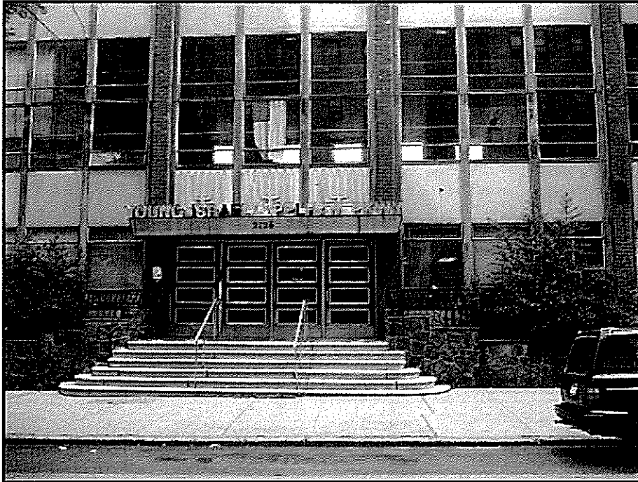
Photo 3 – Barnes Avenue entrance to the existing building on the site
