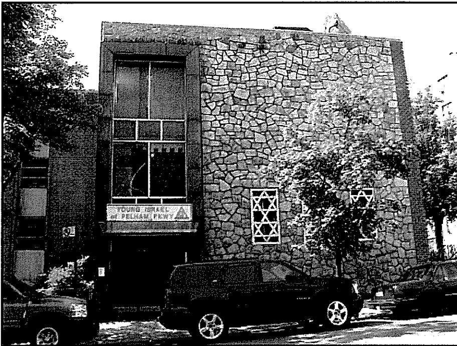
Photo 2 – Existing building at 2126 Barnes Avenue, looking south on Lydig Avenue
