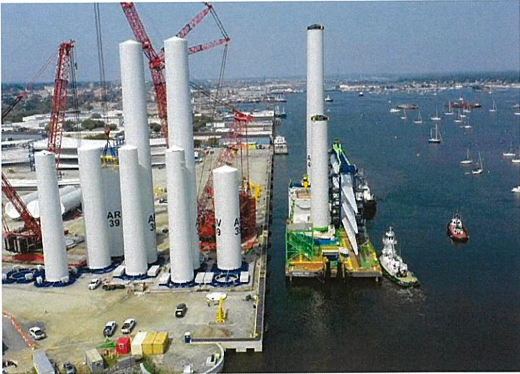
New Bedford Marine Commerce Terminal, New Bedford, MA
