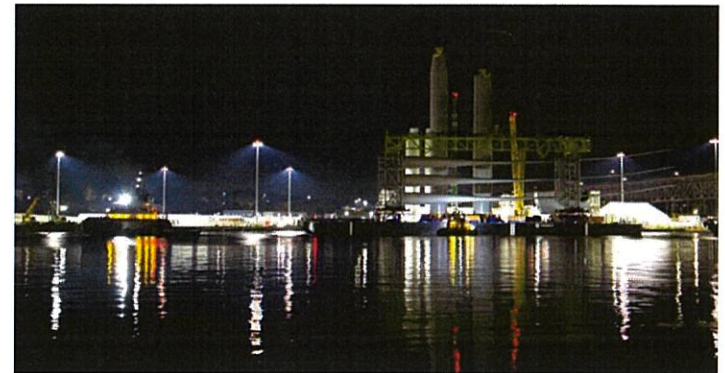
Nighttime Operations at New London State Pier
