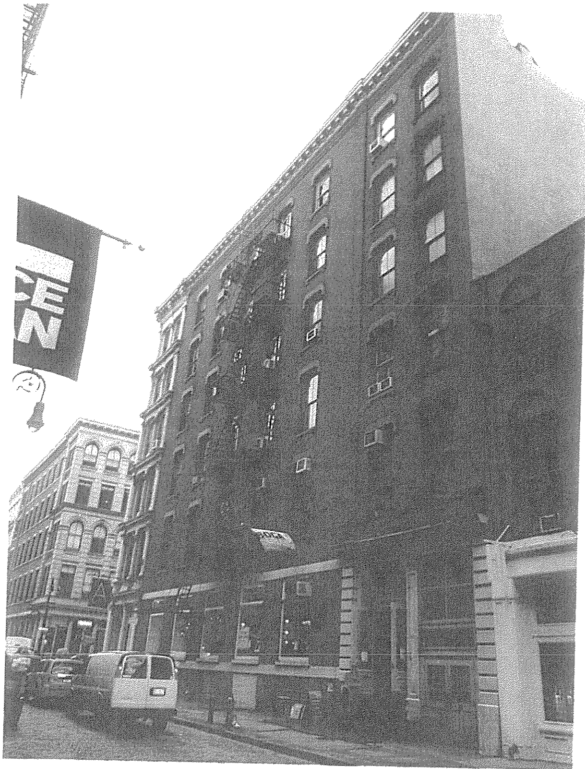
GREENE STREET FACADE
