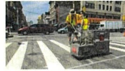
200M linear ft of markings
