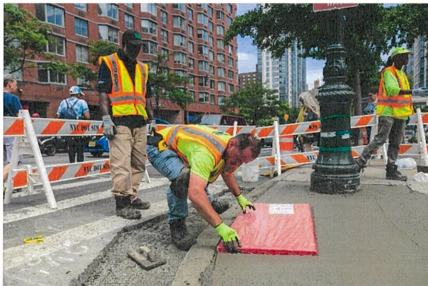
Accessible Pedestrian Signal and Pedestrian Ramp Installations
