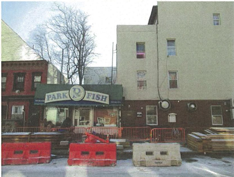
9. View of the Project Area facing south from Park Avenue.
