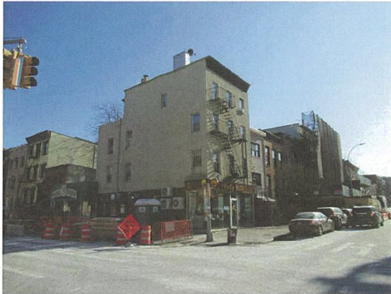
7. View of the Project Area facing southeast from the intersection of Park Avenue and Franklin Avenue.
