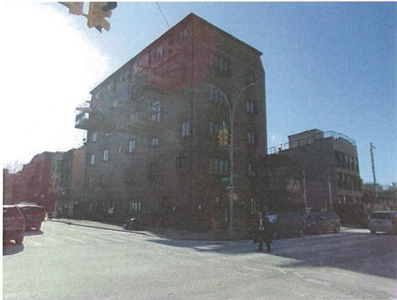
1. View of the Project Area facing southwest from the intersection of Park Avenue and Franklin Avenue.
