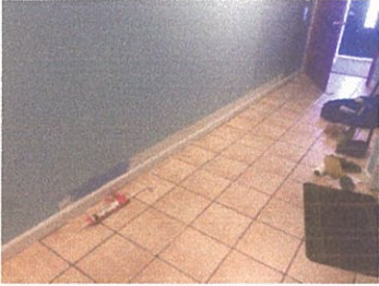
radiators gone February 3, 2016 at 2:35:25 PM
