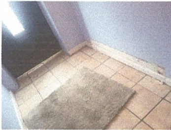
removed entrance radiator February 4, 2016 at 9:37:53 AM
