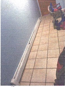
hallway radiator August 4, 2015 at 11:03:51 AM
