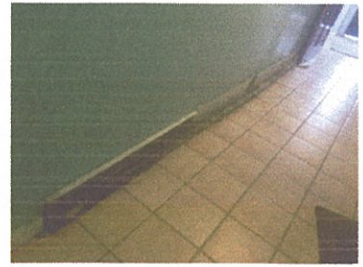
Feb 3 ripped out hallway radiator February 3, 2016 at 10:13:39 AM
