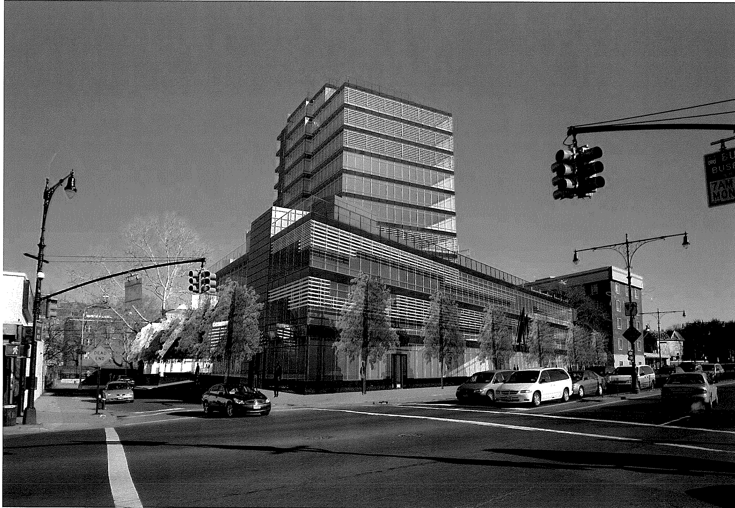
View of completed Project from Fordham Road
