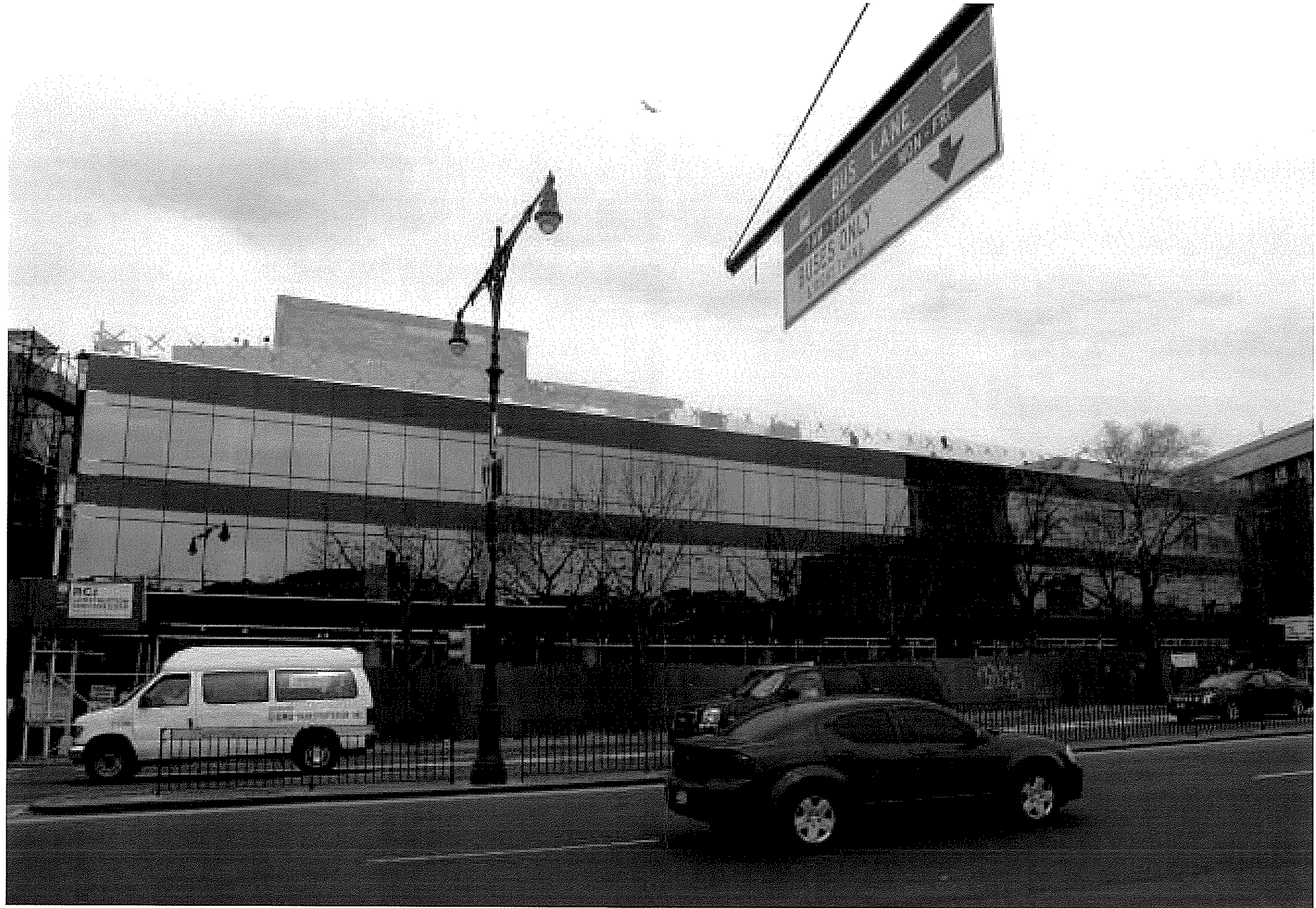
Phase 1 in construction - March 2010
