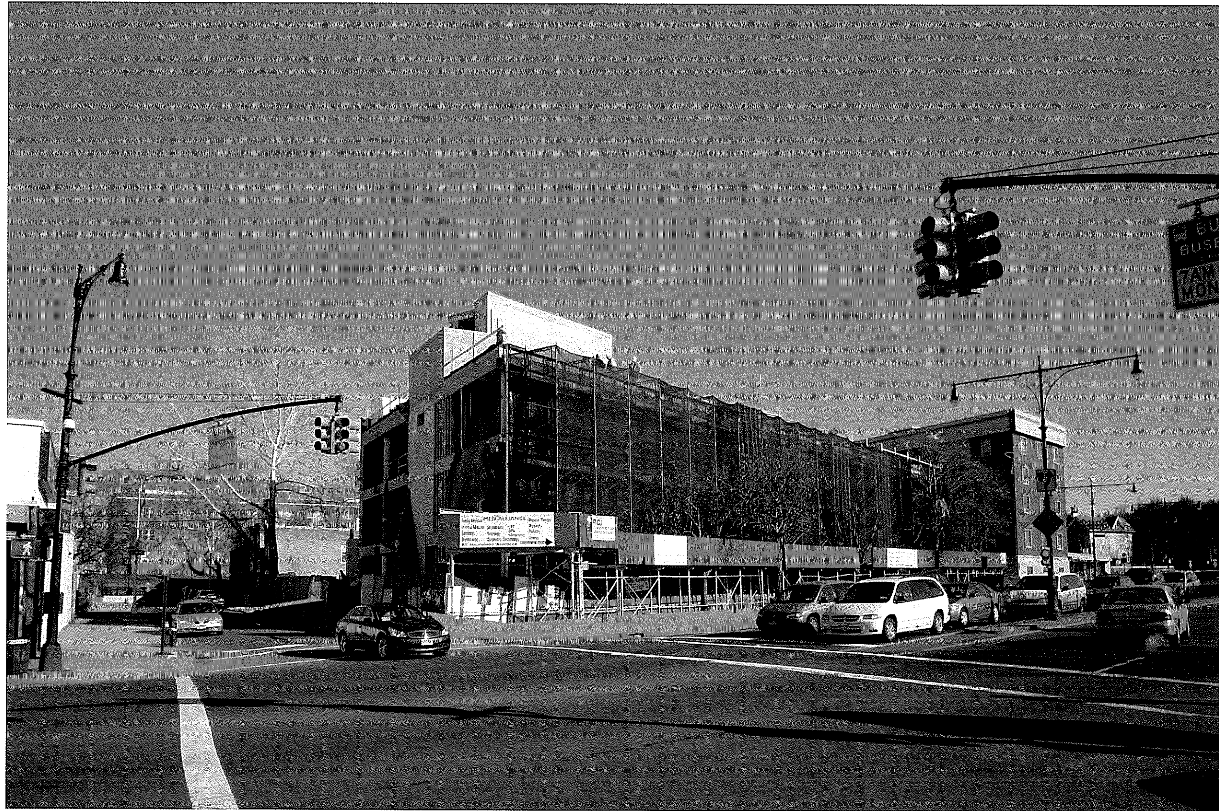
Phase 1 in Construction - January 2010
