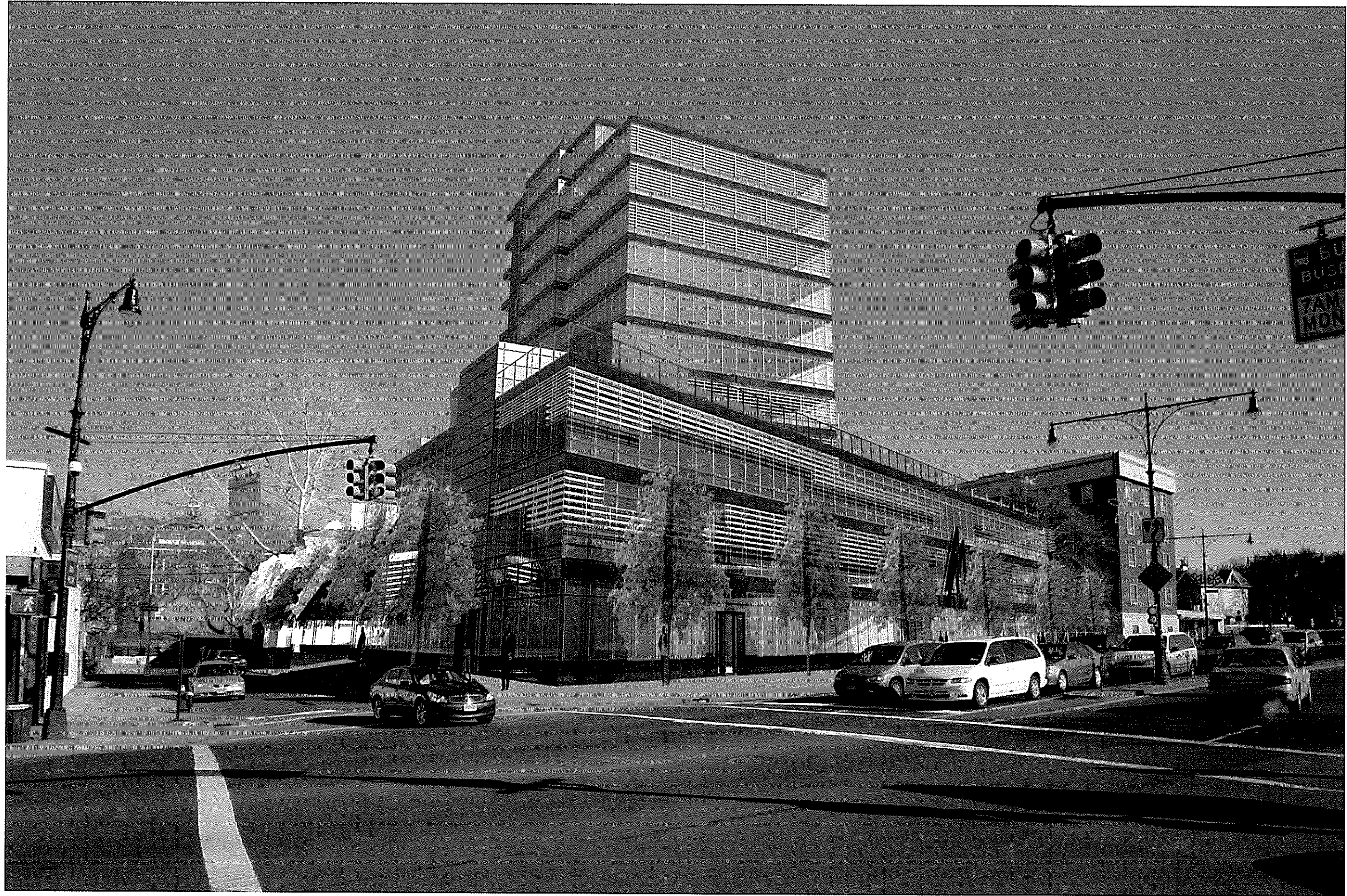
Phases 2 and 3 completed, 10 stories residential above 2- and 3-story base
