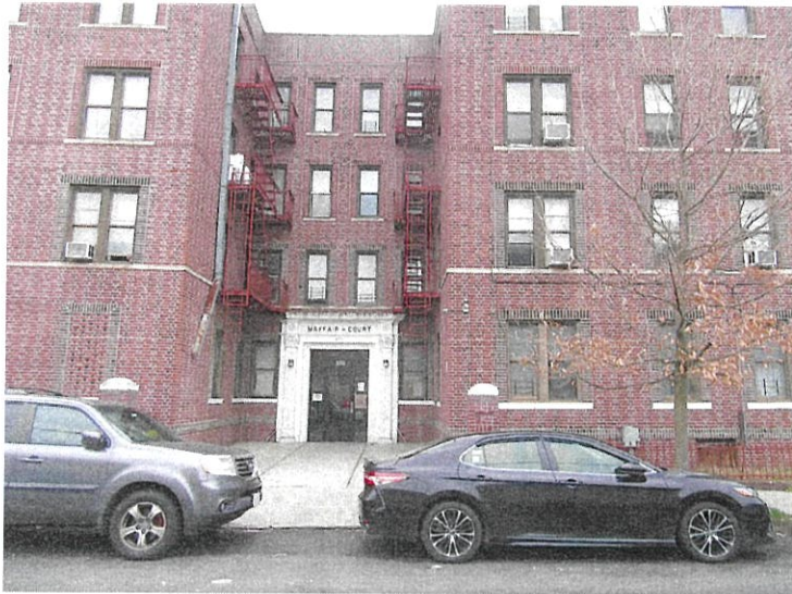
22. View of the Project Area facing east from East 21st Street.
