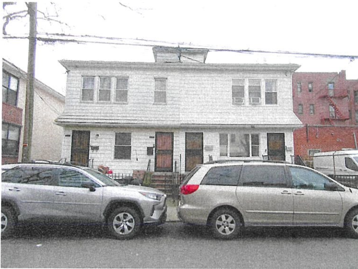
25. View of the Project Area facing east from East 21st Street.
