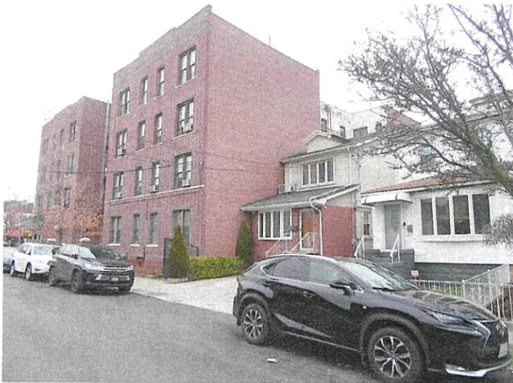
24. View of the Project Area facing northeast from East 21st Street.
