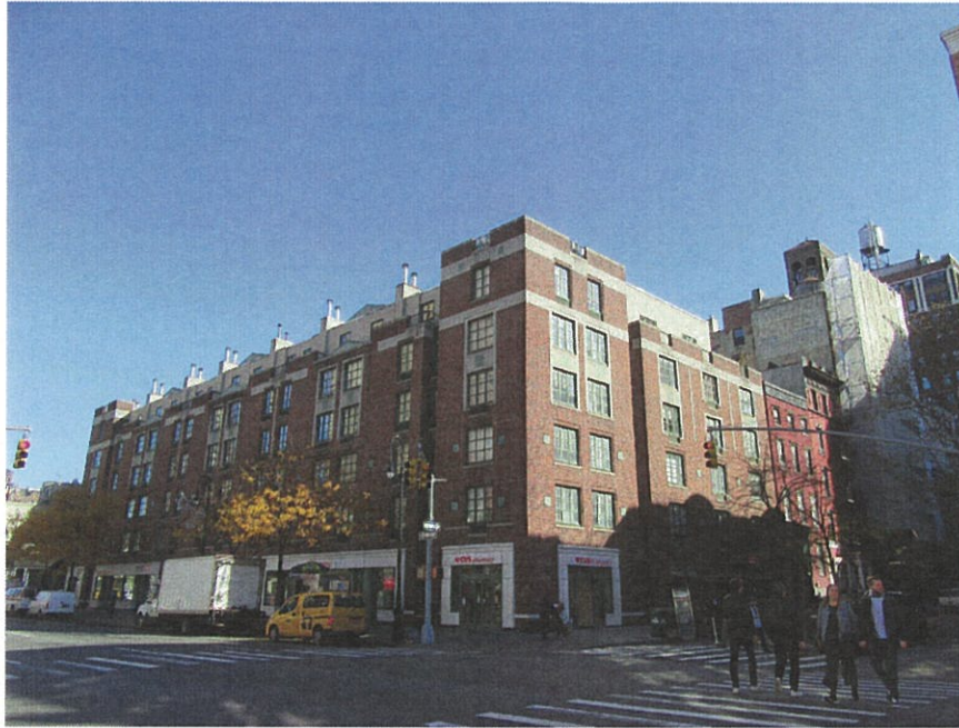
1. View of the Site facing east from the intersection of Washington Place and Avenue of the Americas.
