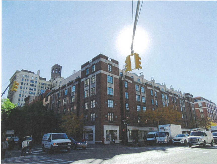
4. View of the Site facing south from the intersection of Avenue of the Americas and Waverly Place.
