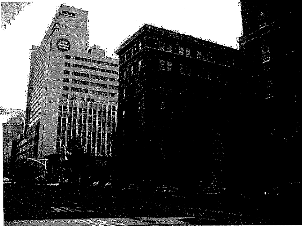
(2) Psychiatric Building with NYU Medical Center and Office of the Chief Medical Examiner to the north.
