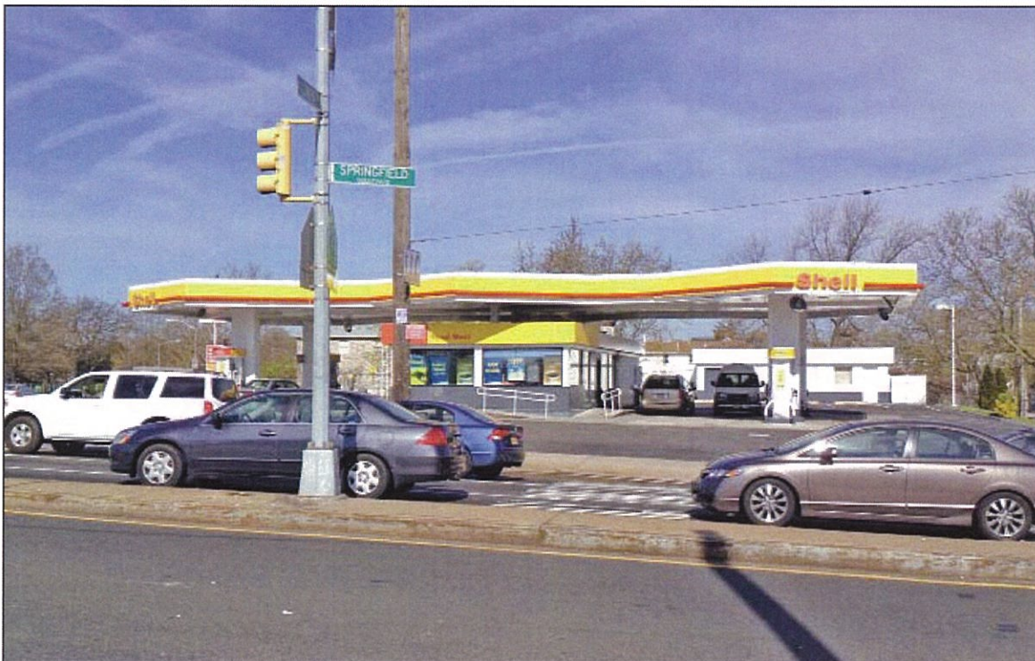
7. A Shell gas station and food mart located across Springfield Boulevard, west of the area to be demapped.
