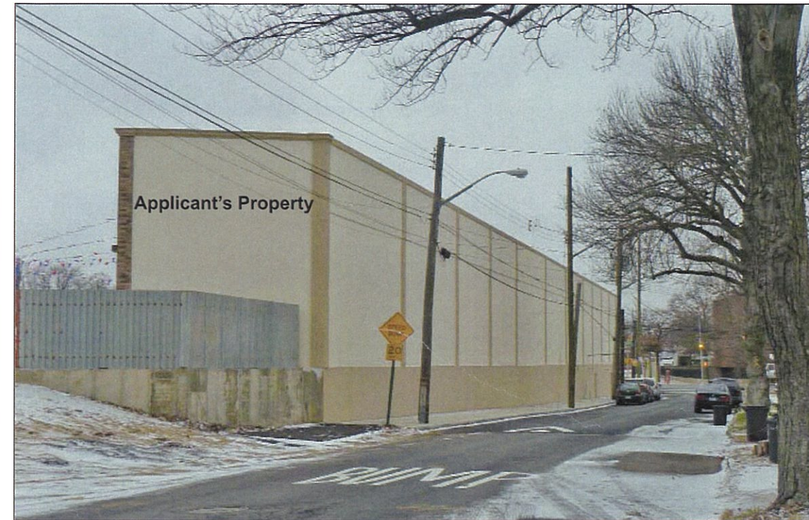
2. Rear view of the commercial uses on the applicant's property on 144th Avenue.
