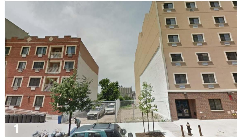
PHOTO #1 : PROJECT SITE - LOOKING WEST
