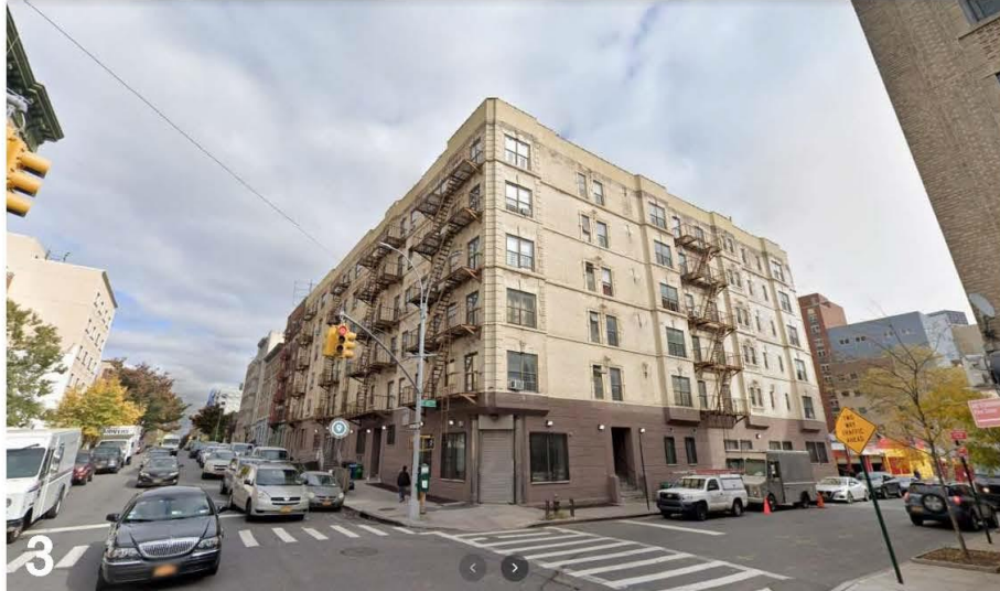
PHOTO #3 : PROJECT SITE - LOOKING NORTH-EAST FROM THE INTERSECTION OF WASHINGTON AVE AND E 167TH ST
