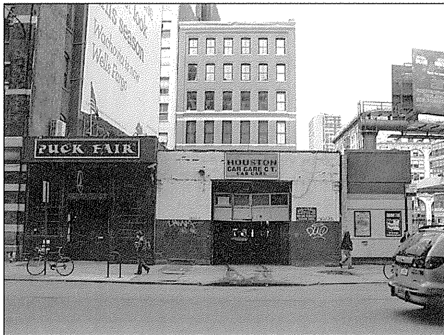
Adjacent one-story non-historic buildings
