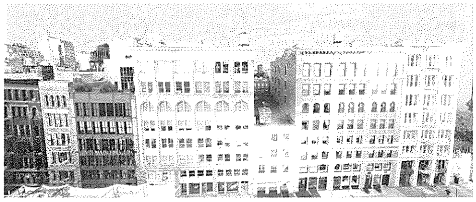
S - W - N VIEW AT PENTHOUSE LEVEL FACING WEST
