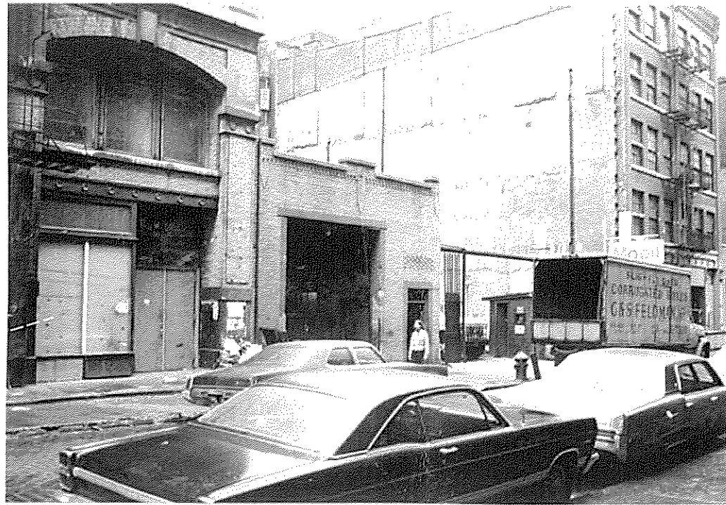
LPC DESIGNATION PHOTO; 1972
