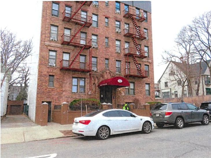
12. View of the Project Area facing west from Ovington Avenue.
