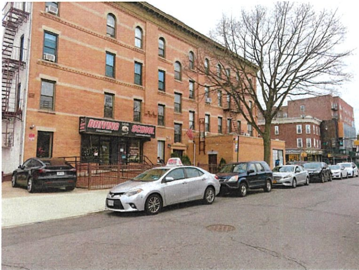
7. View of the northeast side of Ovington Avenue facing northeast from the Development Site.
