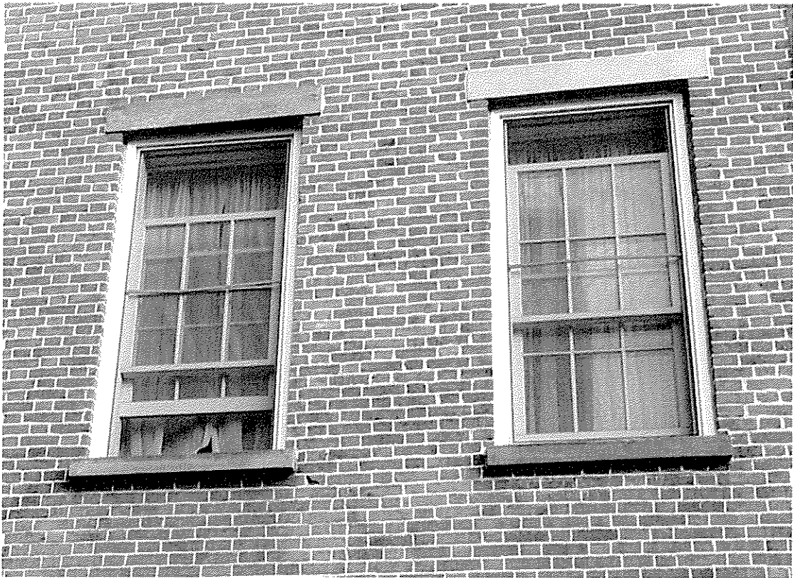
34 Dominick Street LP 2481 Altered lintel – precast concrete
