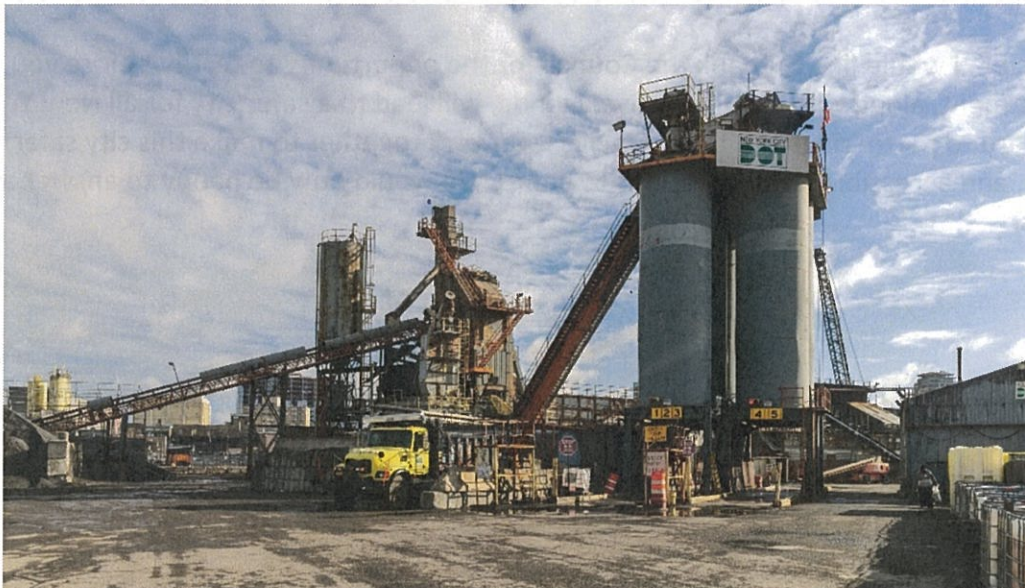
Harper Street Asphalt Plant
