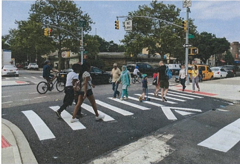
Raised Crosswalk at East 5 th Street and Fort Hamilton Parkway, Brooklyn
