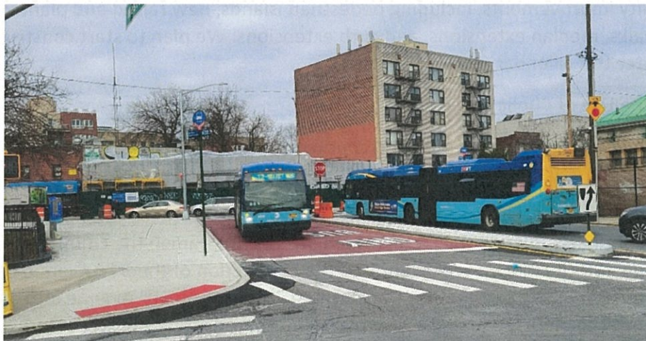
Pelham Bay Park Station Transit Improvements
