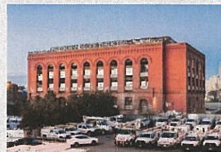
Brooklyn Rapid Transit (B.R.T.) Central Powerhouse
