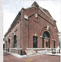
Gowanus Canal Flushing Tunnel Pump House
