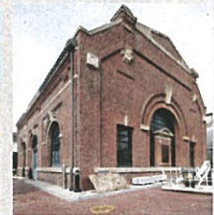
Gowanus Canal Flushing Tunnel Pump House
