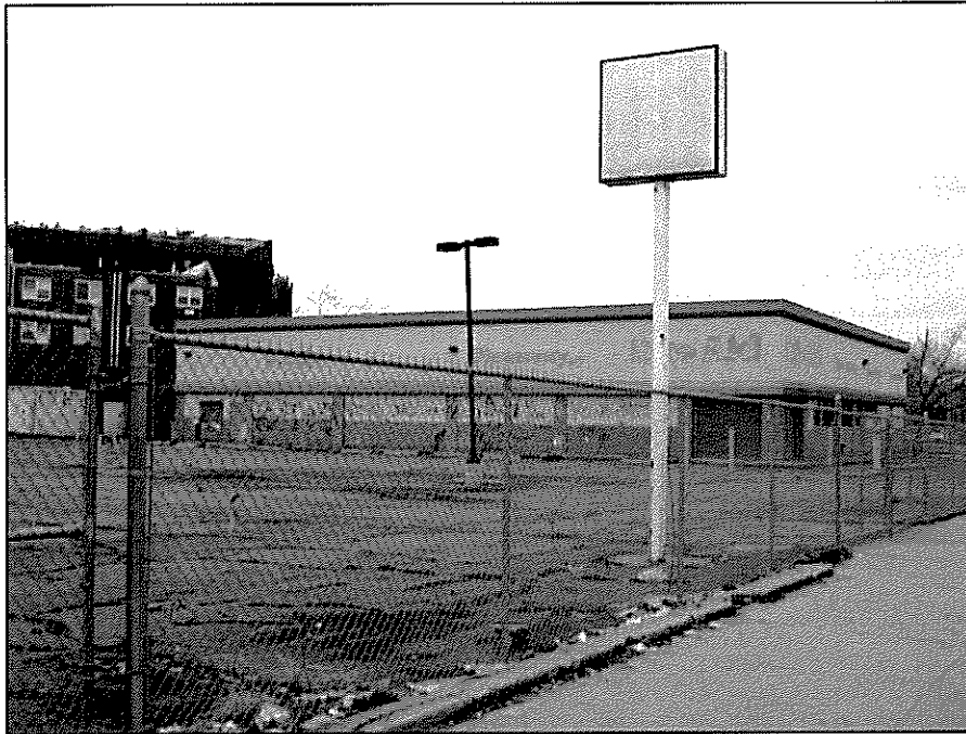
Photograph 1 – Vacant Building on Project Site
