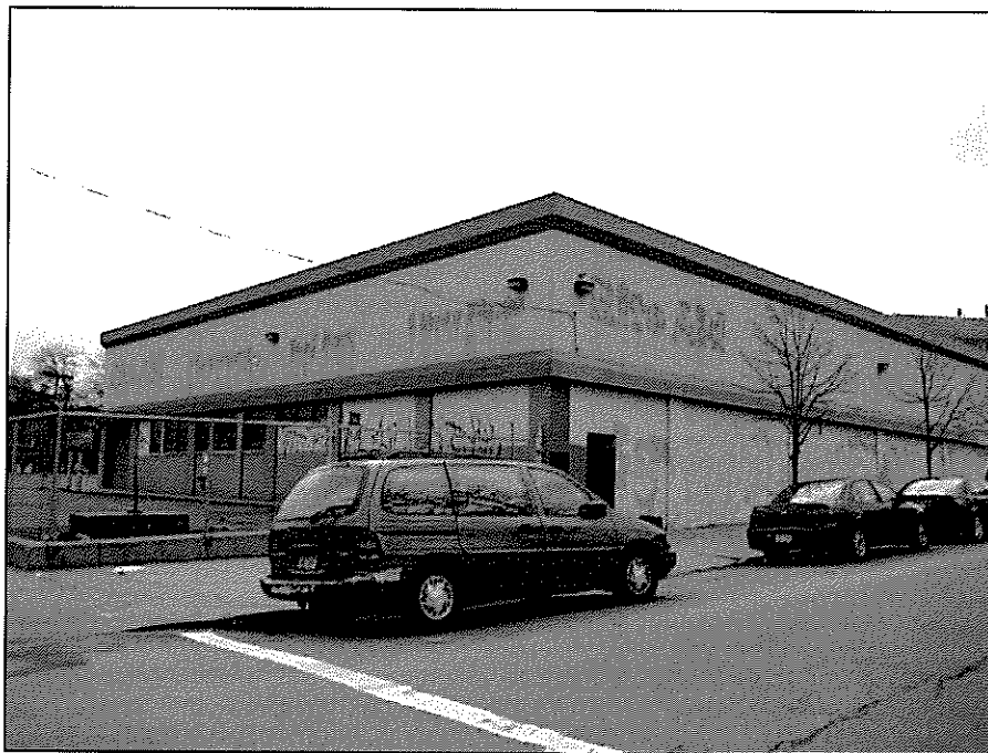
Photograph 3 – Additional View of Vacant Building on Project Site
