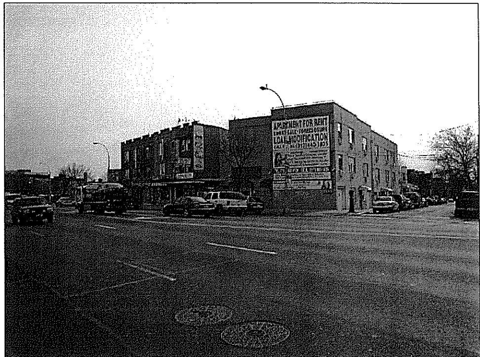
View southeast from 109th Street to south side of Northern Boulevard 14
