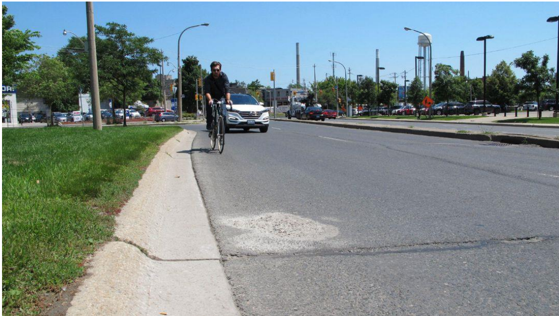
Hardened piles of cement dropped on the road by overloaded cement trucks, such as this one on Eastern Ave., [Toronto], can be hard for cyclists to avoid without swinging into fast-moving traffic. Photo and quote by Jack Lakey, The Toronto Star
