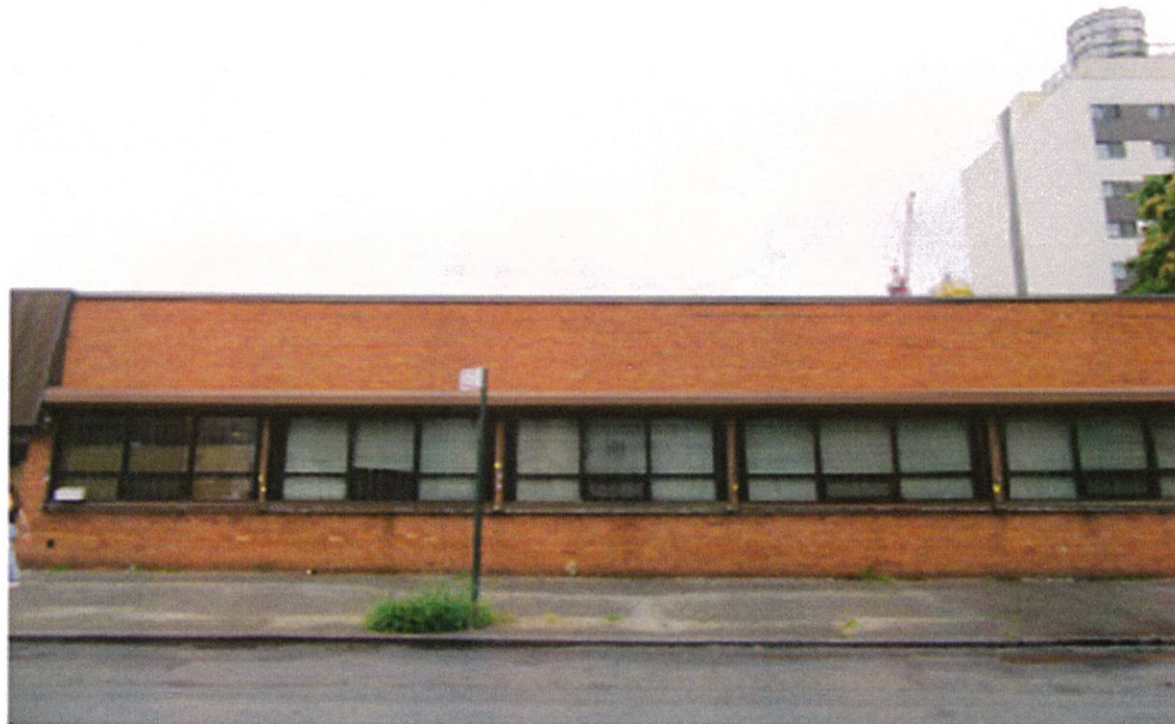
6. View of the Development Site facing southeast from Crescent Street.
